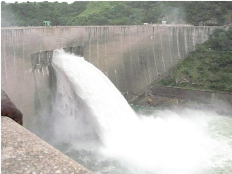
Figure 1: Photo of Kariba dam showing 1 of the 6 sluices spilling
