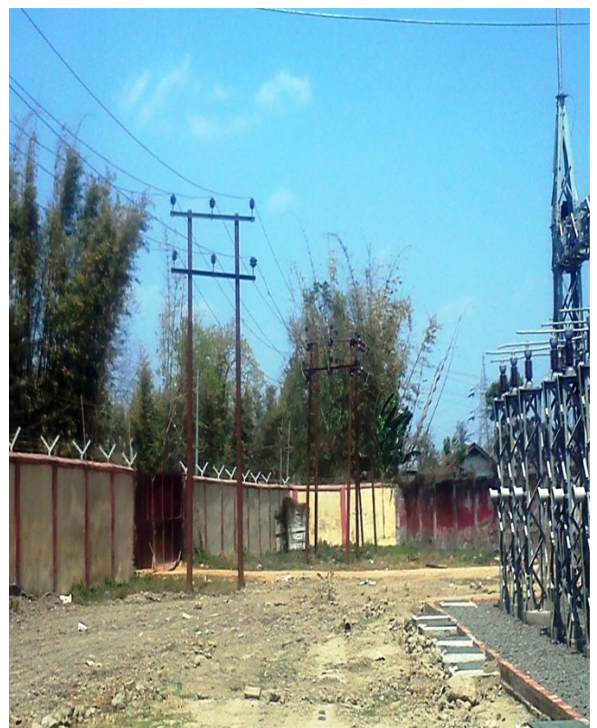
33 kV (H Pole) line inside substation
