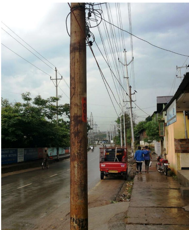
33 kV line inside city area of Assam
