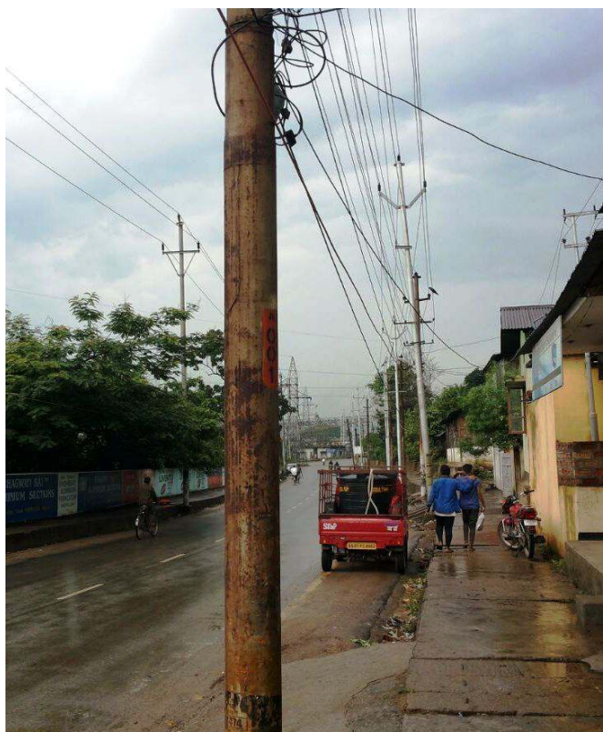
33 kV line inside city area of Assam
