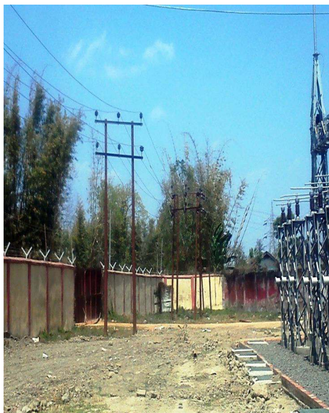
33 kV (H Pole) line inside substation
