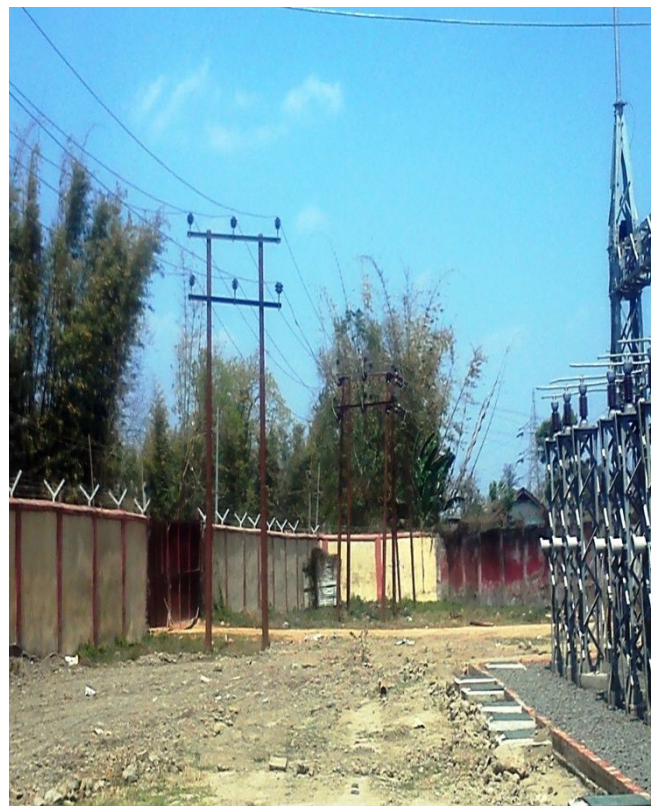
33 kV (H Pole) line inside substation
