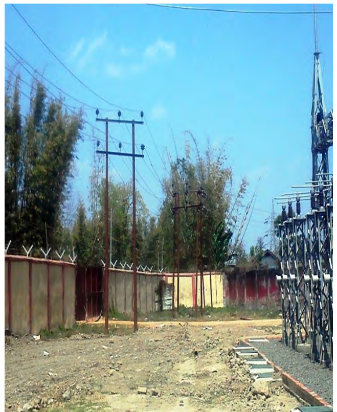
33 kV (H Pole) line inside substation
