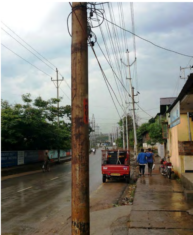
33 kV line inside city area of Assam
