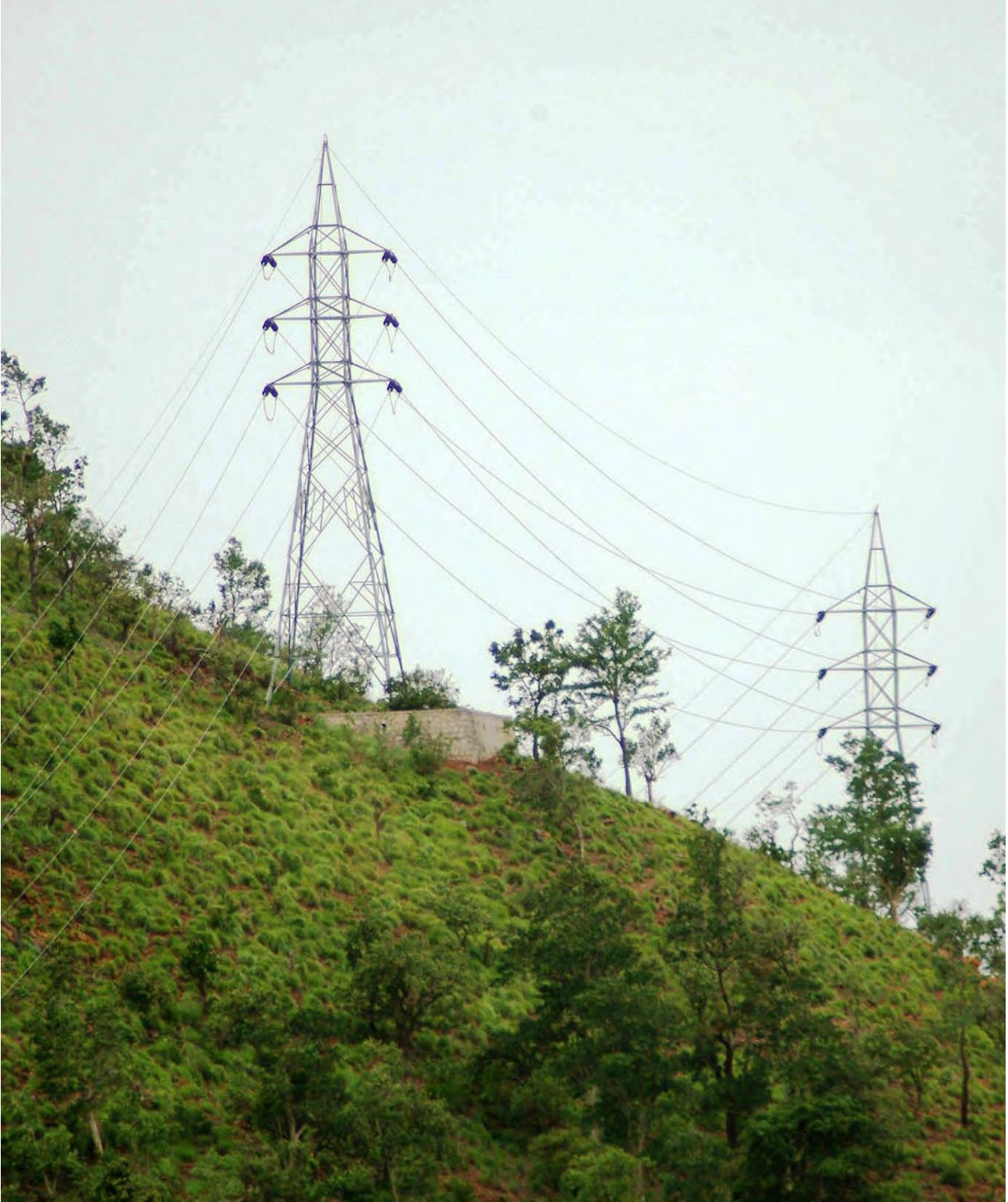
Fig. -1 132 kV line depicting actual position along with RoW and extent of damage
