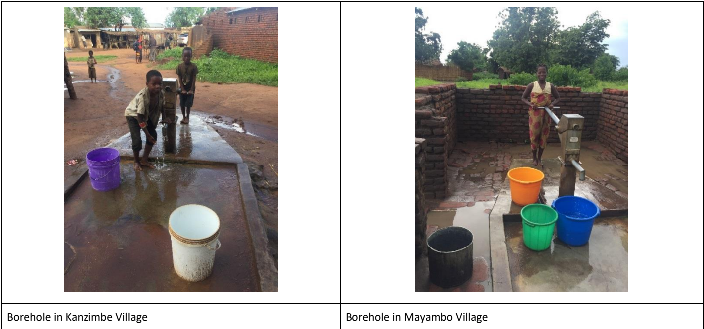
Figure 19: Boreholes in Kanzimbe and Mayambo Villages
