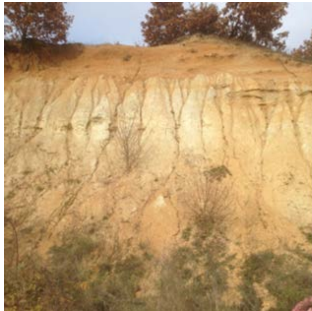
Figure 40: Surface wash-off in cohesionless sediments occurring at section Km 16+000 – Km 21+000
