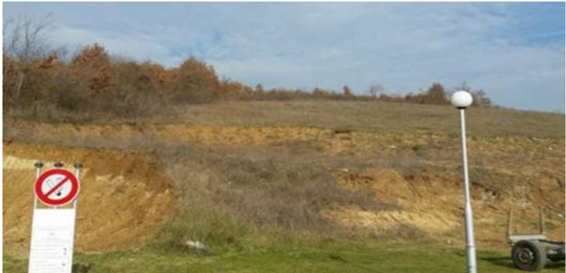
Figure 21: Km 15+000: Area of a 17-18m cut
