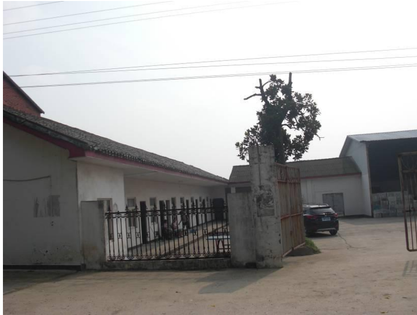
Figure 2-7 Green Waxing Plant
