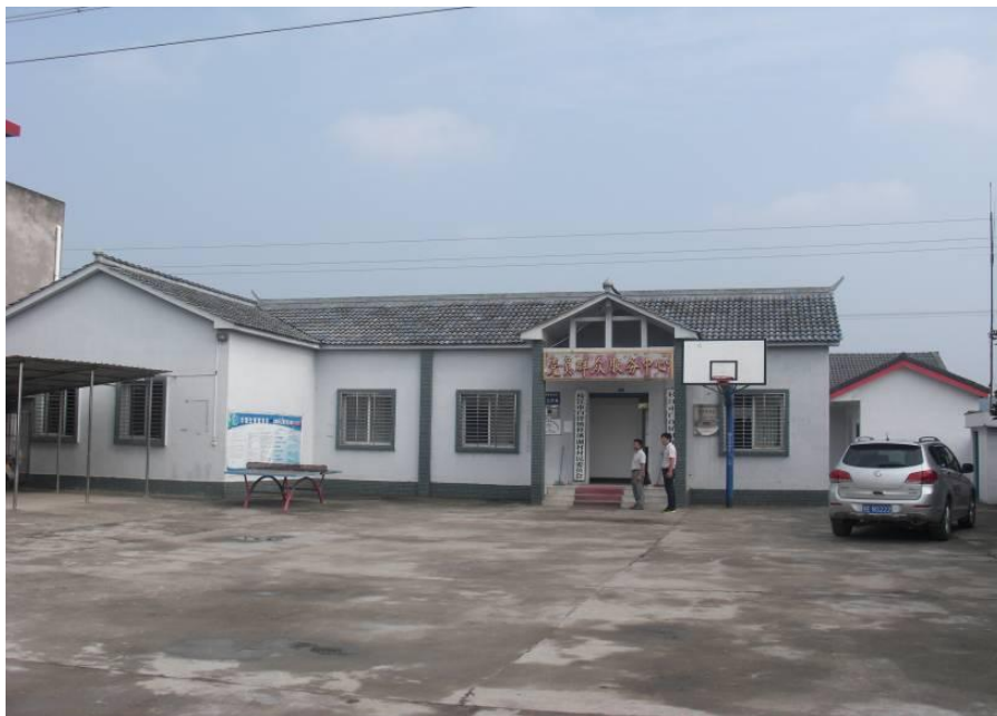
Figure 2-6 Guixihu Village Committee building to be demolished
