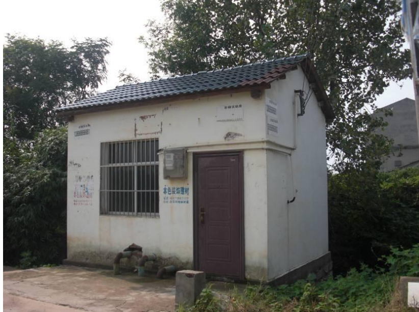
Figure 2-10 Pressurization room of Baiyang Water Plant
