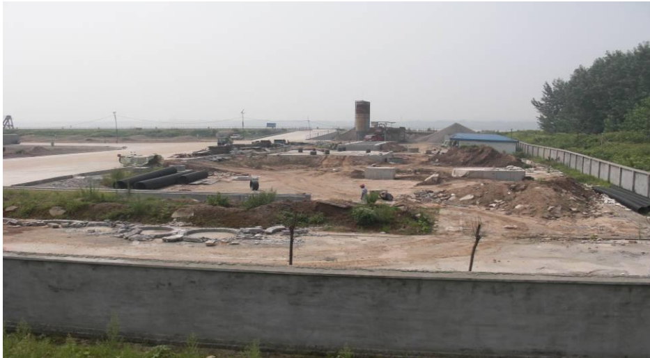
Figure 1 Baiyang Port Operation Area Phase I project under construction
