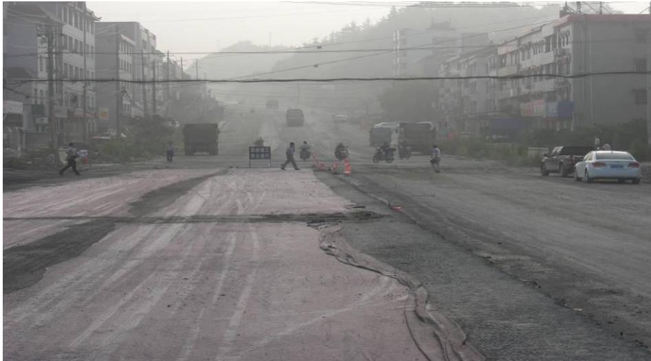
Figure 2 Baiyang Logistics Park – Taibaochang Section of New National Highway 318 Rerouting Project under construction
