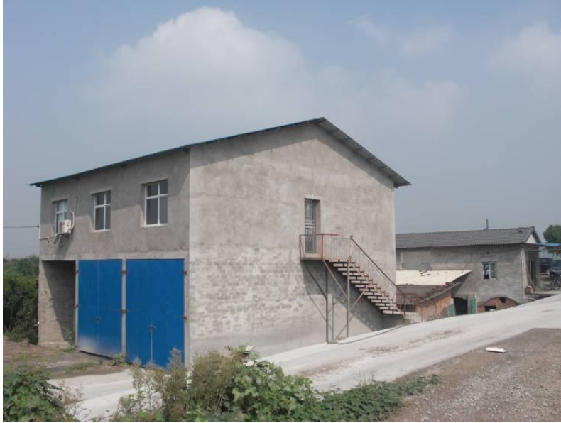
Figure 2-12 Management building of Sand and Stone Factory
