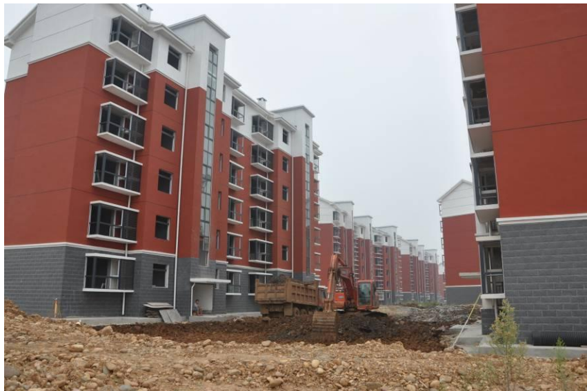
Figure 6-1 Nearly-completed resettlement houses of Baiyang Industrial New Town Resettlement Community Phase II
