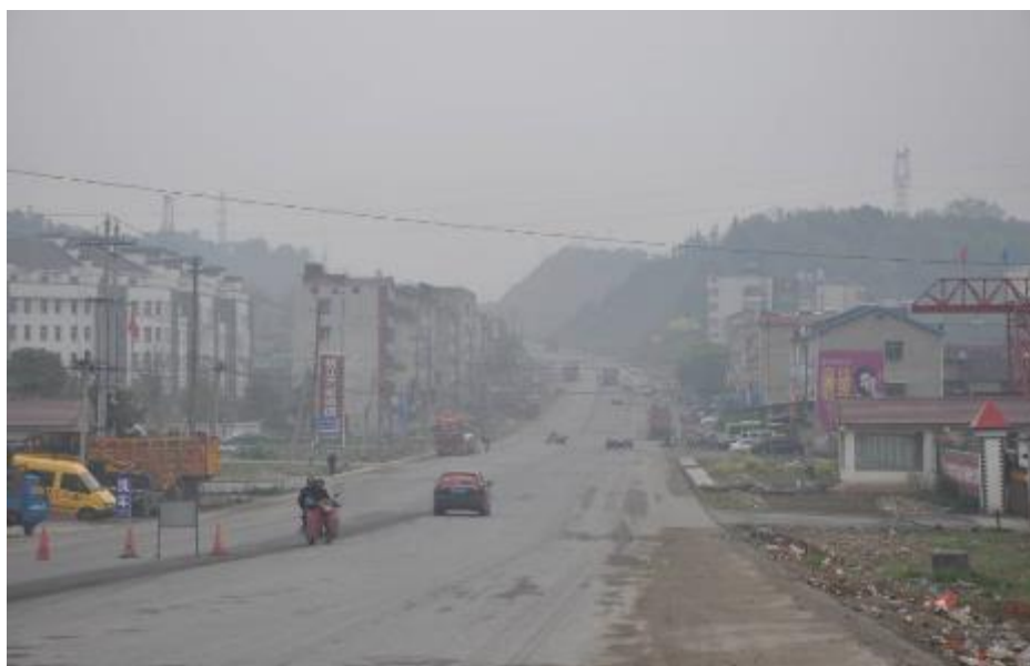
Figure 9-2 No traffic lights at intersections
