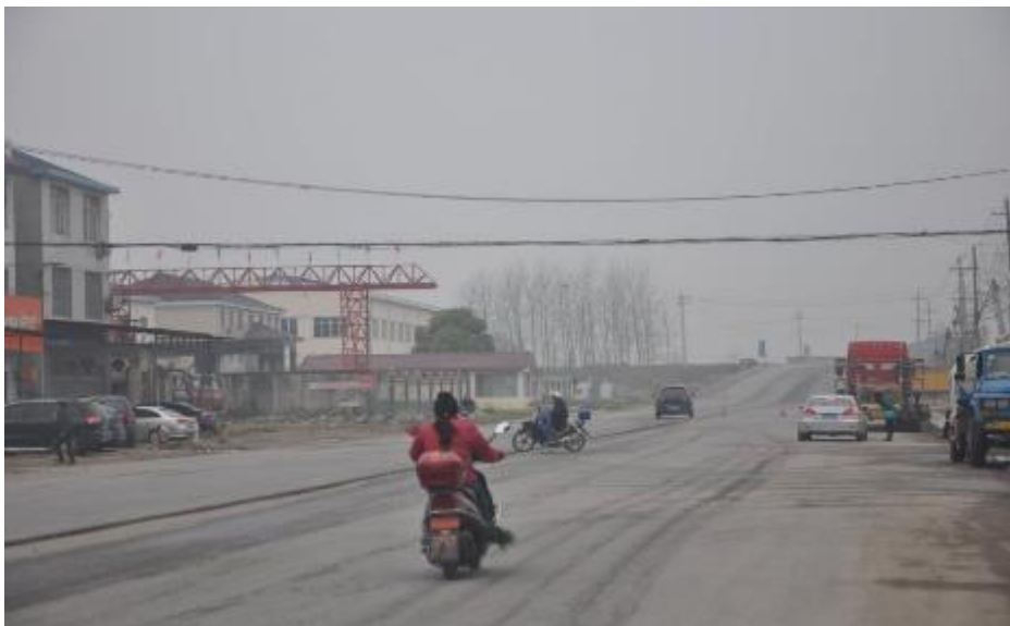
Figure 9-1 Mixed traffic on national road G318
