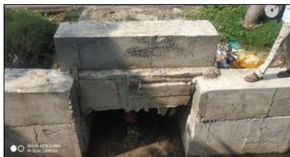
Slab Culvert at km 4/000
