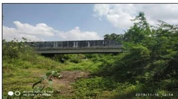
Minor Bridge at Km 2/200 (SH 04)
