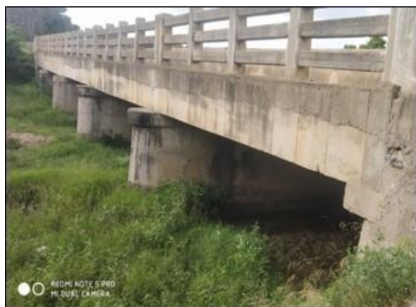
Minor Bridge at km 9/135
