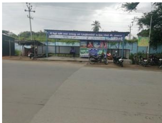
Bus Shelter on RHS at km 13/010
