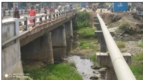
Minor Bridge at km 159/215
