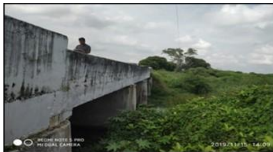
Minor Bridge at Km 8/940 (SH 116)
