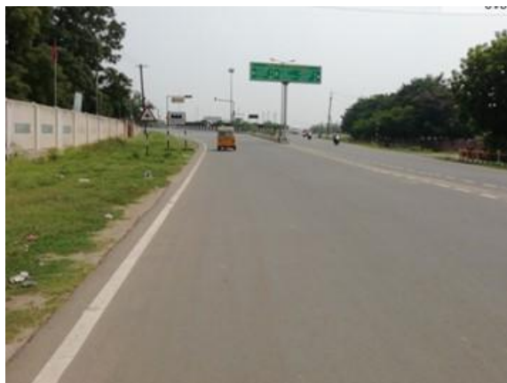
Good pavement condition at km 1/200
