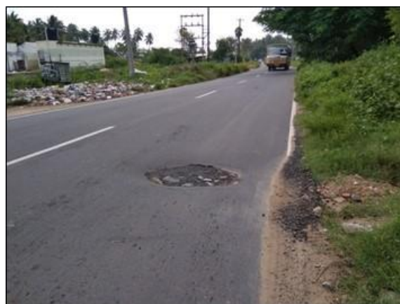
Pothole at km 11/600
