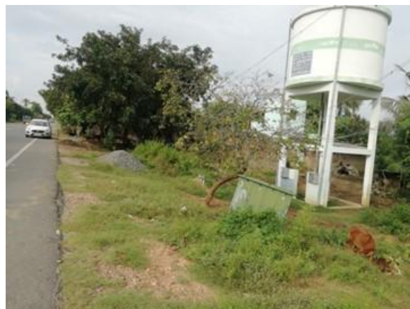
Overhead tank on LHS at km 12/020
