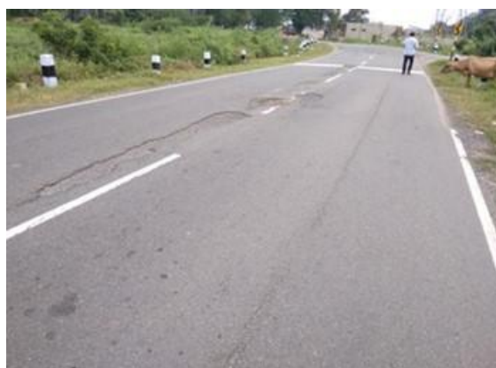
Potholes at km 86/550
