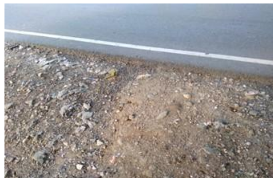
Edge drop at km 2/600
