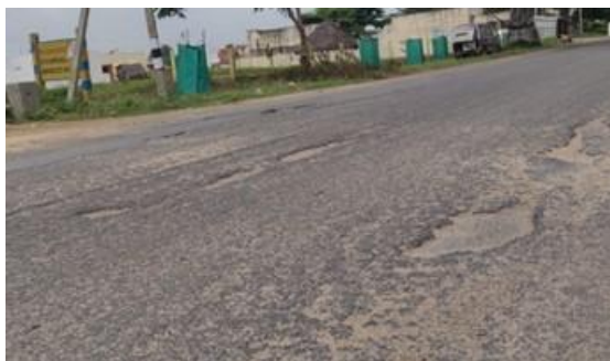
Very poor pavement condition at km 6/300
