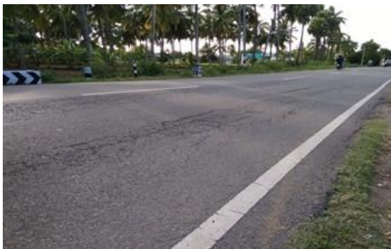
Alligator cracks at km 2/000
