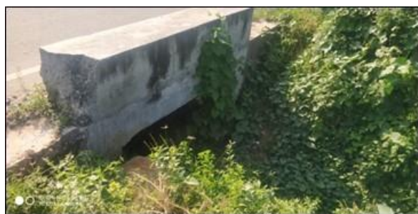
Box Culvert at Km 3/700
