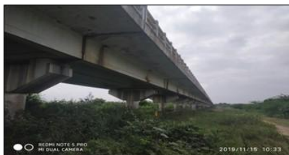
Major Bridge (Palar River ) at km 4/876
