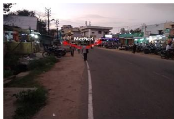
The endpoint of SH 222 (km 14/600)
