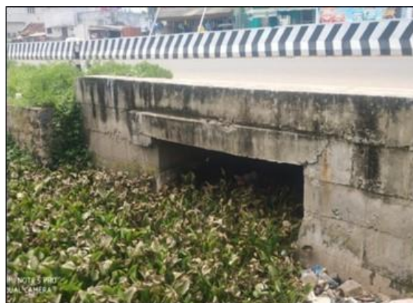
Slab Culvert at km 0/569
