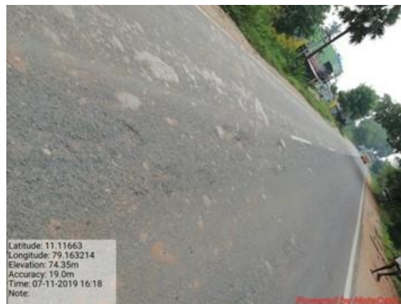
Raveling at km 10/600
