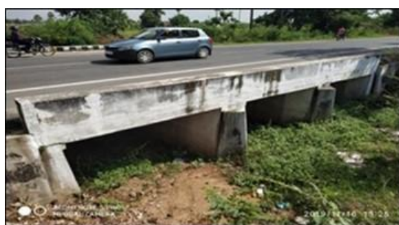
Minor Bridge at km 4/400
