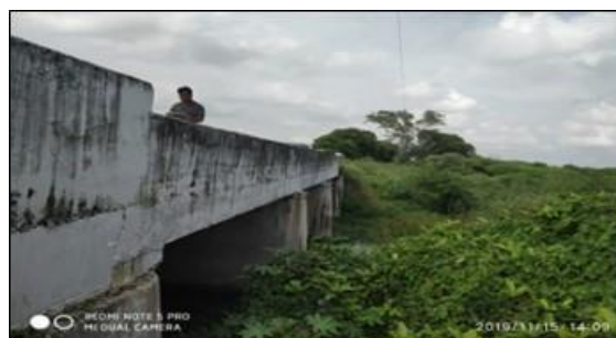
Minor Bridge at km 8/940
