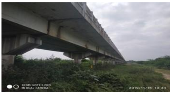
Major Bridge at Km 4/876 (SH 116)
