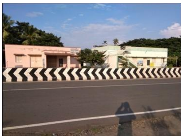
Hospital on LHS at km 3/810
