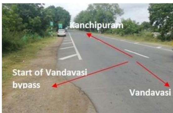
Vandavasi bypass at km 36/560 (SH 116) - Start Point
