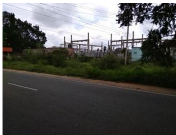
Substation RHS at km 89/180
