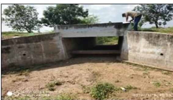
Slab Culvert at km 3/900
