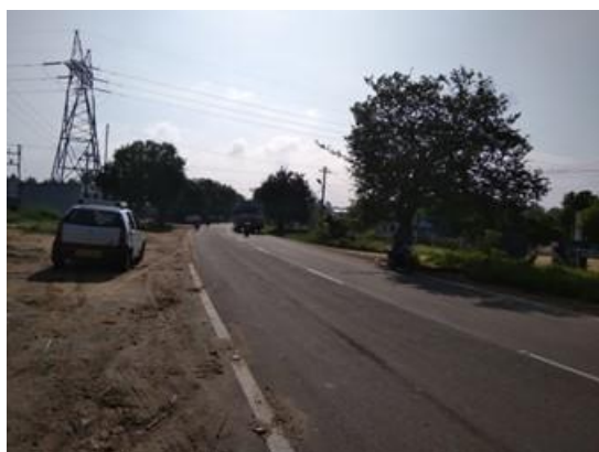
Longitudinal cracking at km 154/100
