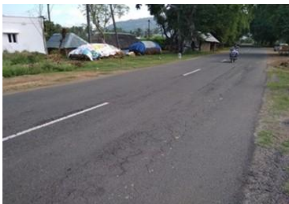
Alligator cracks at km 82/600
