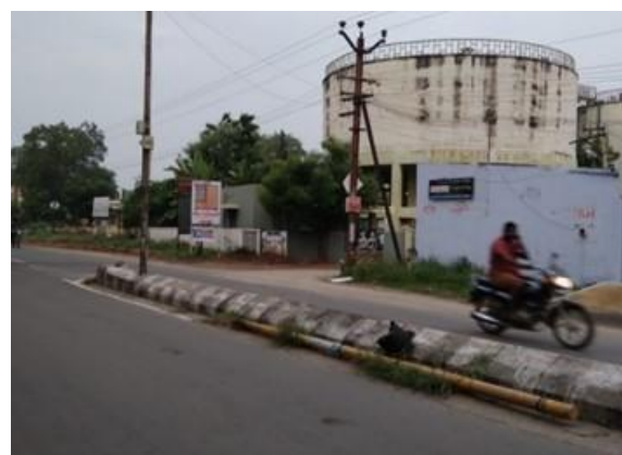
Overhead tank on RHS at km 1/060
