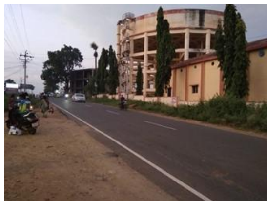
Overhead Tank on RHS at km 14/140
