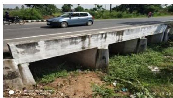
Minor Bridge at Km 4/400 (SH 04)
