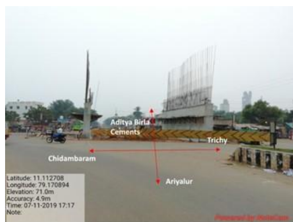
The endpoint of SH 139 (km 11/600)
