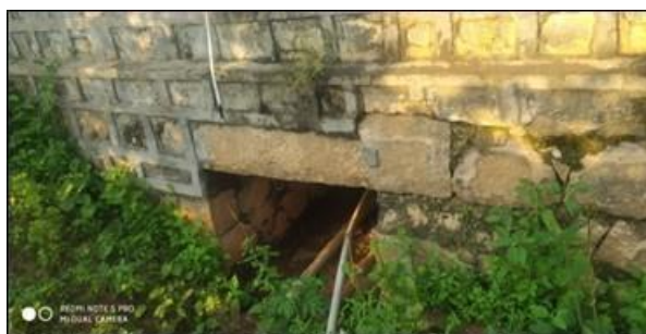
Cut Stone Slab Culvert at Km 6/900
