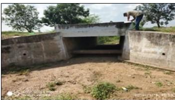
Slab Culvert at km 3/900
