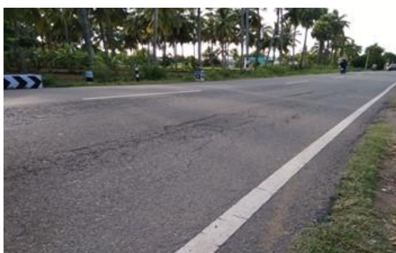
Alligator cracks at km 2/000
