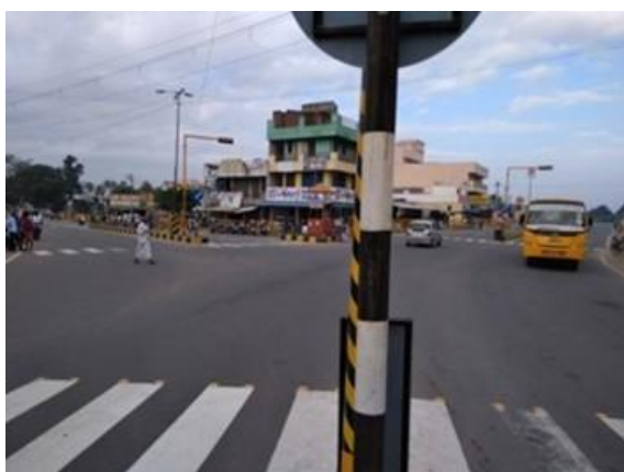
Major Intersection (SH 79) at km 0.000
