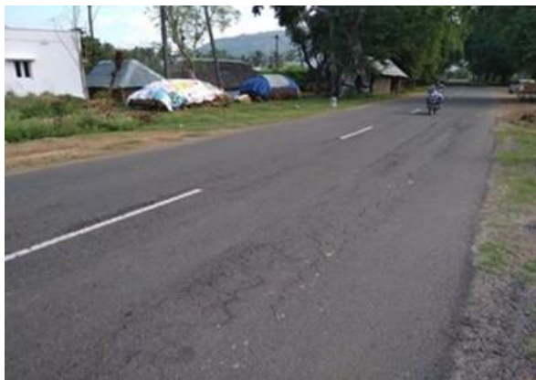
Alligator cracks at km 82/600
