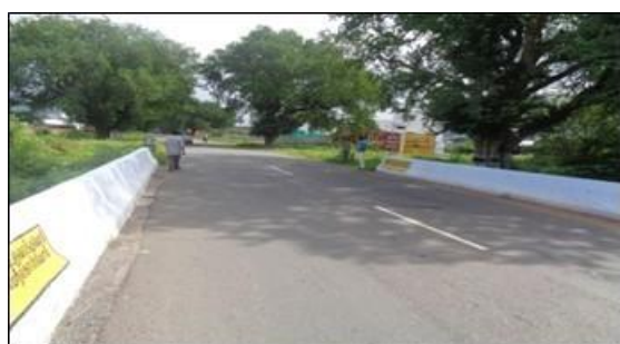
Minor Bridge at km 82/447
