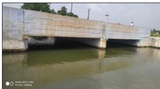
Minor Bridge at km 14/700
