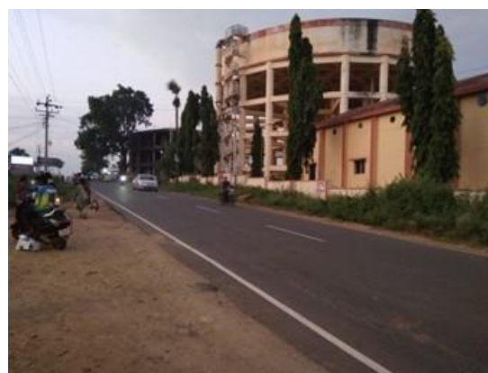
Overhead Tank on RHS at km 14/140
