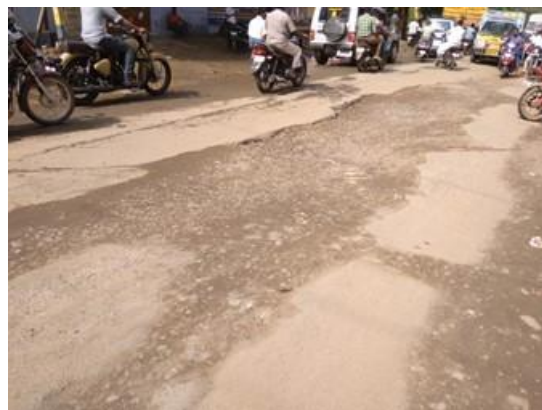
Distressed pavement at km 161/200
