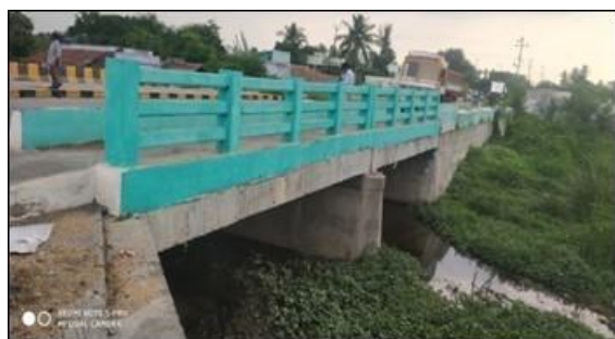
Minor Bridge at km 4/585
