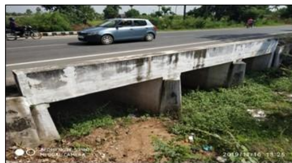
Minor Bridge at Km 4/400 (SH 04)
