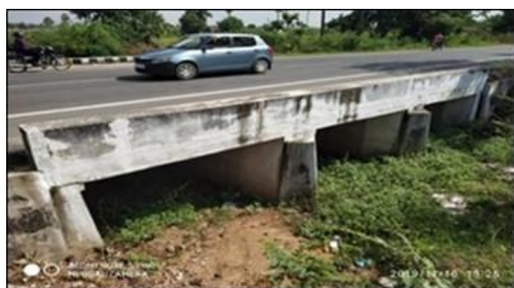
Minor Bridge at km 4/400
