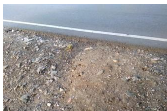
Edge drop at km 2/600
