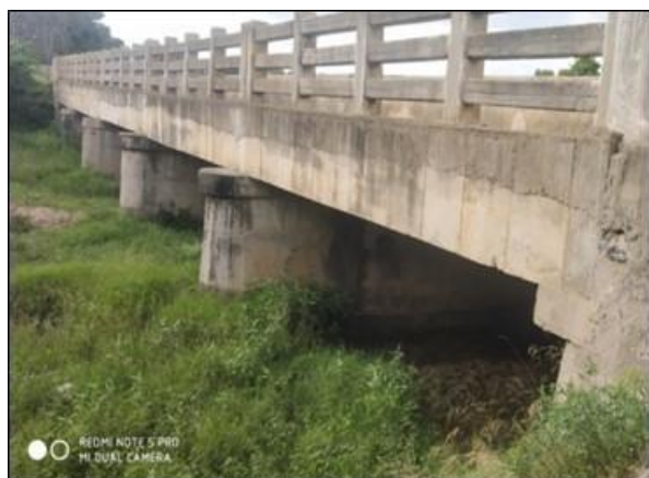
Minor Bridge at km 9/135
