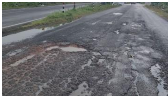
Very poor pavement condition at km 9/000
