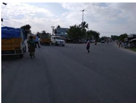
Major Intersection (SH-86) at km 0/000
