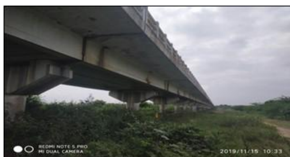
Major Bridge (Palar River ) at km 4/876
