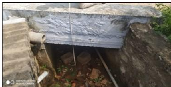
Slab Culvert at km 19/000
