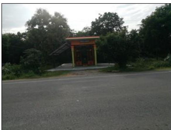
Temple on RHS at km 12/500
