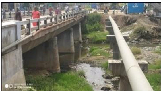
Minor Bridge at km 159/215
