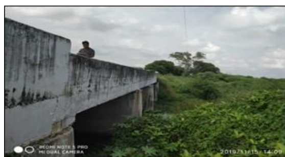
Minor Bridge at km 8/940
