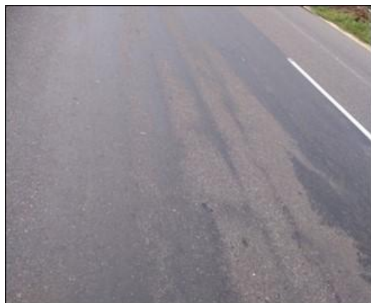
Bleeding at km 16/900
