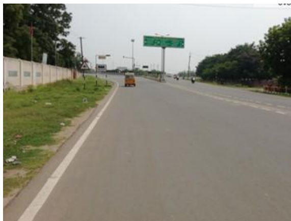
Good pavement condition at km 1/200
