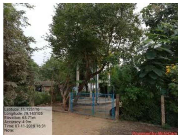
Overhead tank on LHS at km 8/230
