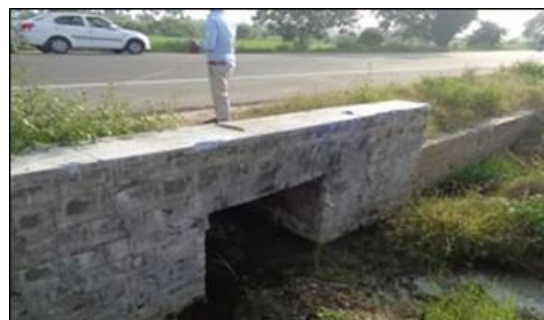
Slab Culvert at km 154/870
