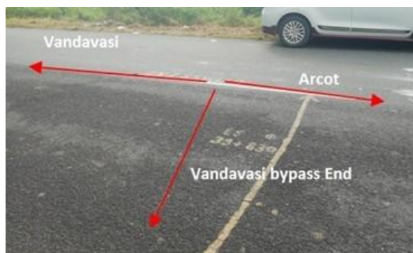
Vandavasi bypass at km 56/100 (SH 05) - End Point
