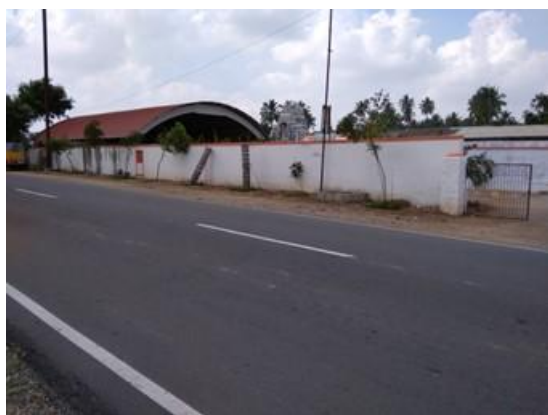
Temple on RHS at km 9/360
