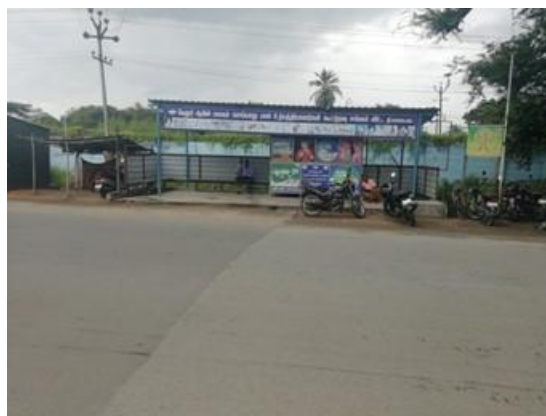
Bus Shelter on RHS at km 13/010
