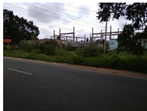
Substation RHS at km 89/180
