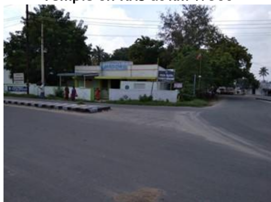
Primary Health Center on RHS at km 13/340
