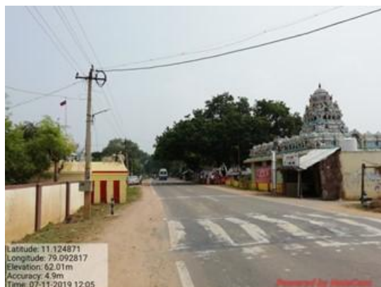
Temple on RHS at km 2/270
