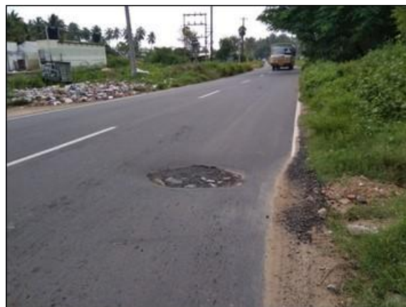
Pothole at km 11/600
