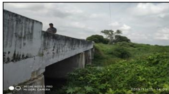
Minor Bridge at Km 8/940 (SH 116)
