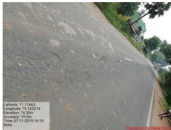
Raveling at km 10/600
