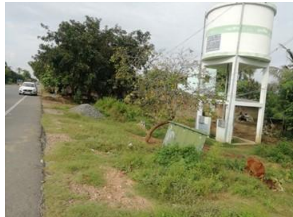
Overhead tank on LHS at km 12/020
