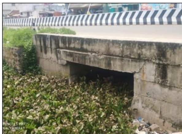
Slab Culvert at km 0/569
