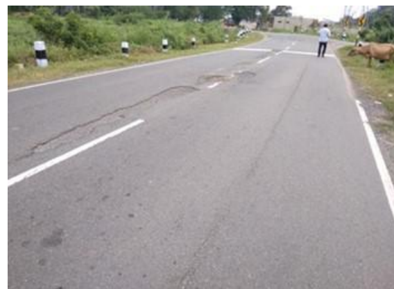
Potholes at km 86/550
