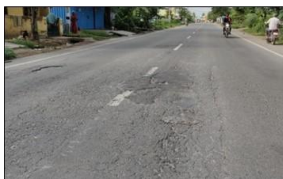
Potholes at km 10/200
