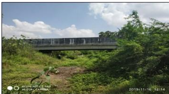
Minor Bridge at Km 2/200 (SH 04)
