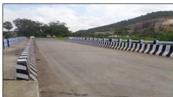
Minor Bridge at km 86/430
