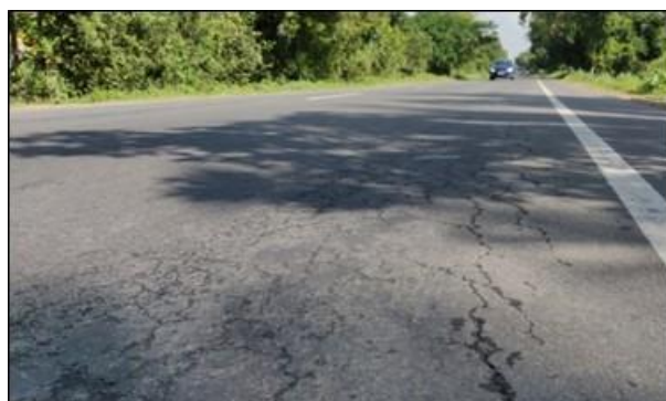
Alligator cracks at km 4/400
