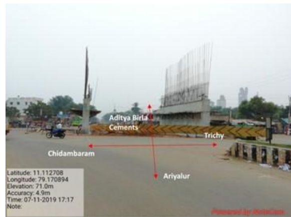
The endpoint of SH 139 (km 11/600)
