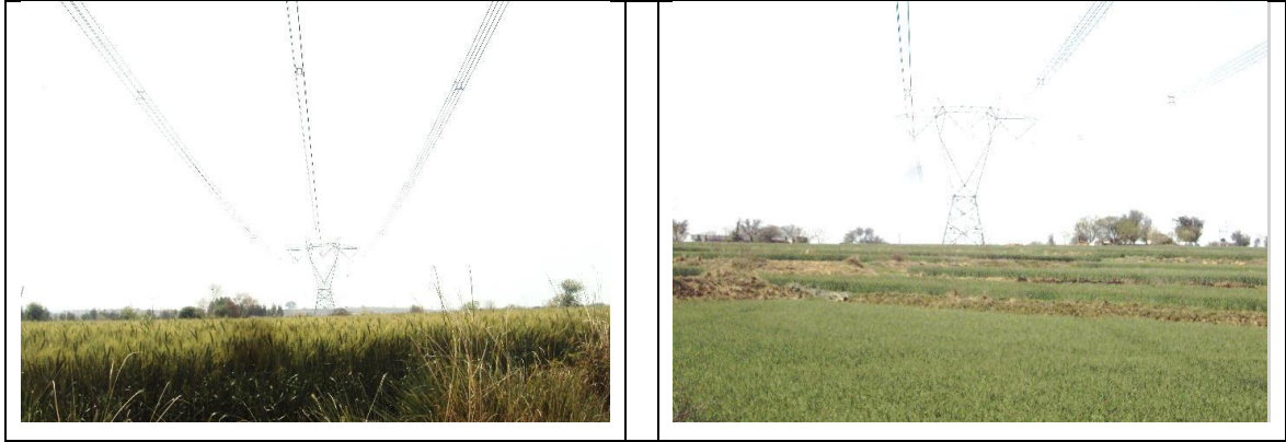
Figure A2.3: Photographs along the Tarbela – Rewat Transmission Line Cultivated land underneath the Tarbela – Rewat line
