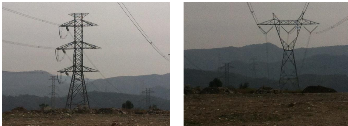
Figure 3.6: Double Circuit Tower and Single Circuit Flat Formation Tower
