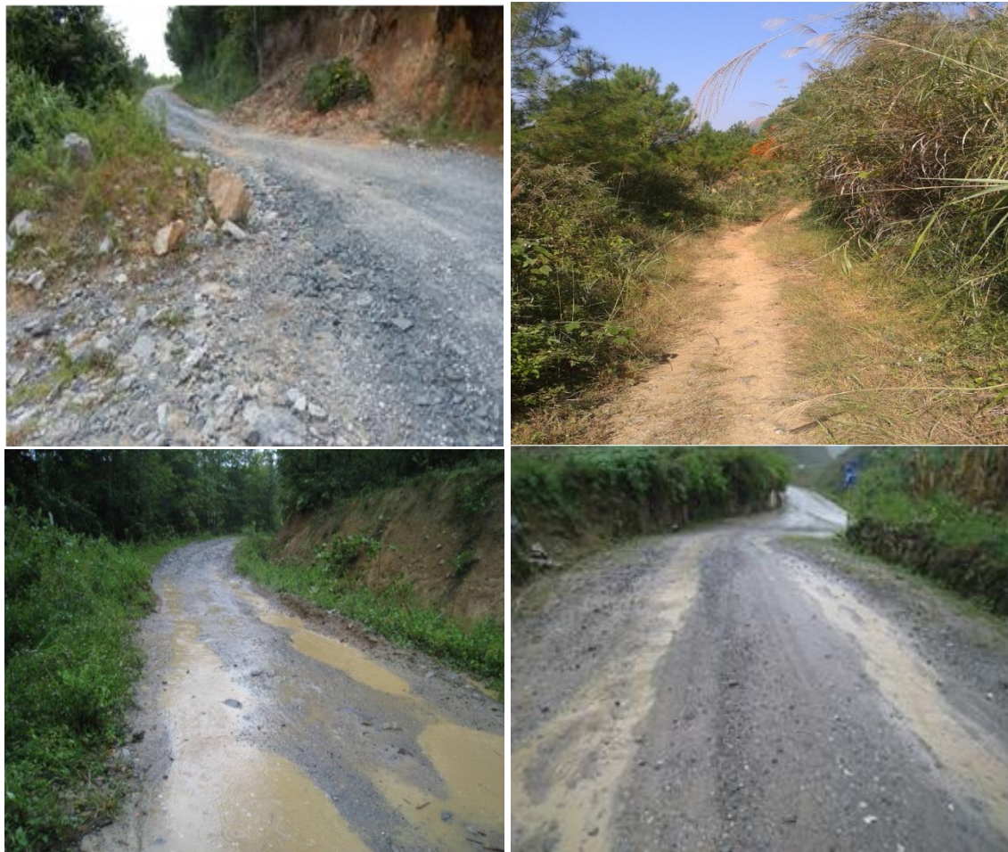
Figure 1-1 Current State of Some Rural Roads in Dejiang and Sinan
