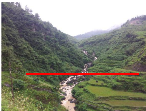
Lengshuiyan Bridge of Changfeng Village
