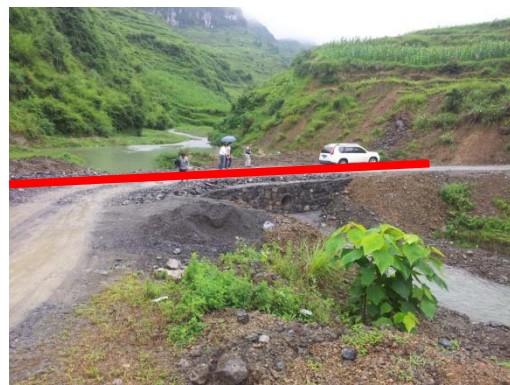
Chuanqian Bridge of Changfeng Village
