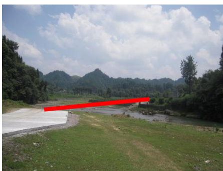
Guanyinyan Bridge of Jiancha Town
