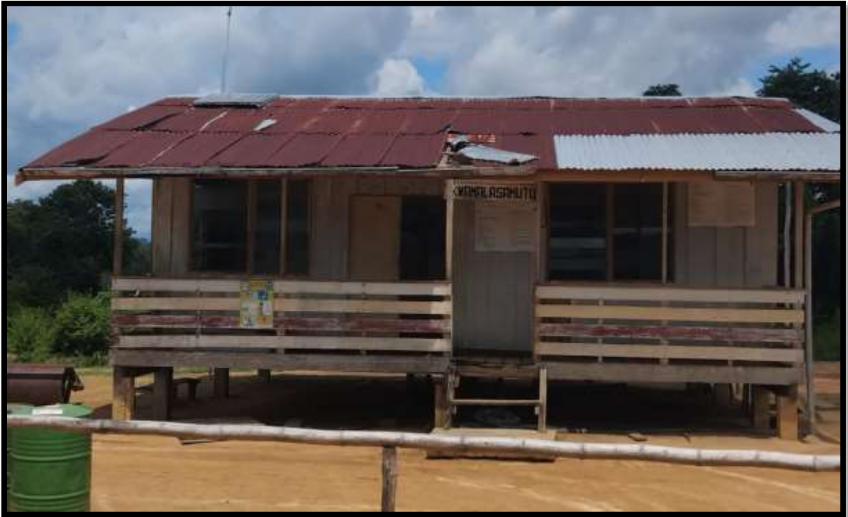
Figure 2. Current office building from the outside
