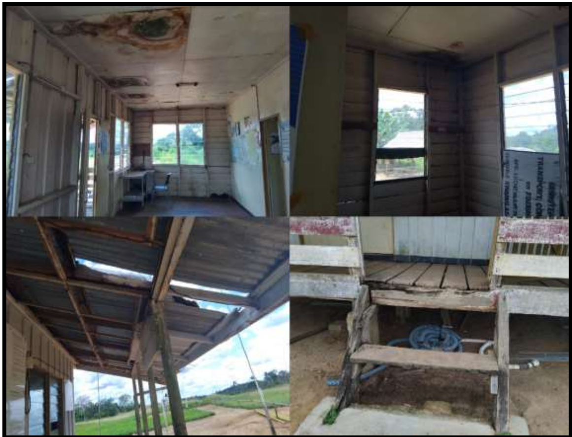
Figure 3. Office Condition (inside and outside)
