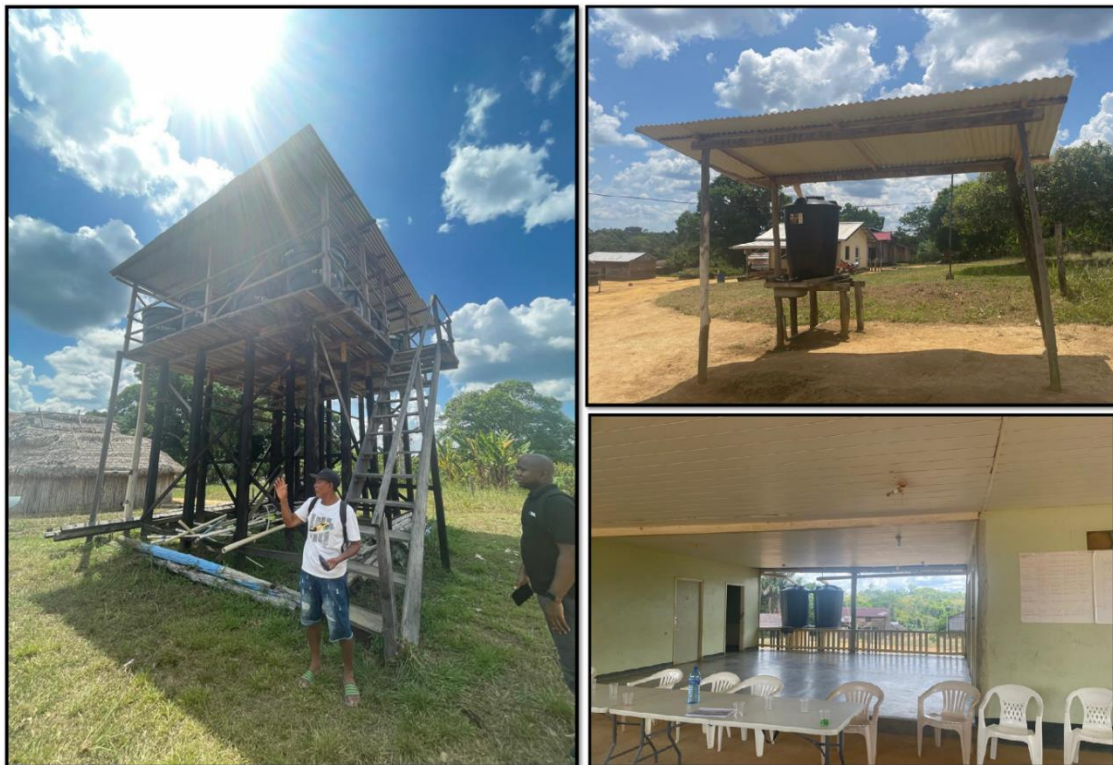
Figure 43. Rain water catchment systems for water. Source: PlanEHS, 2024.
