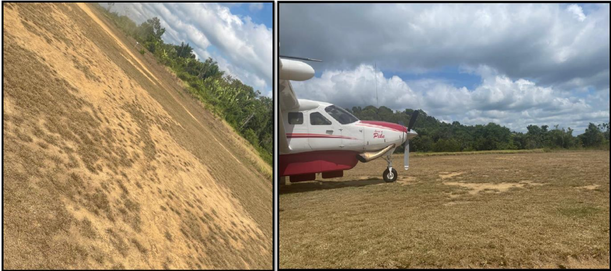
Figure 39. Kwamalasamutu Airstrip conditions: unpaved, uneven, with patches of grass and bare soil. Source: PlanEHS, 2024.
