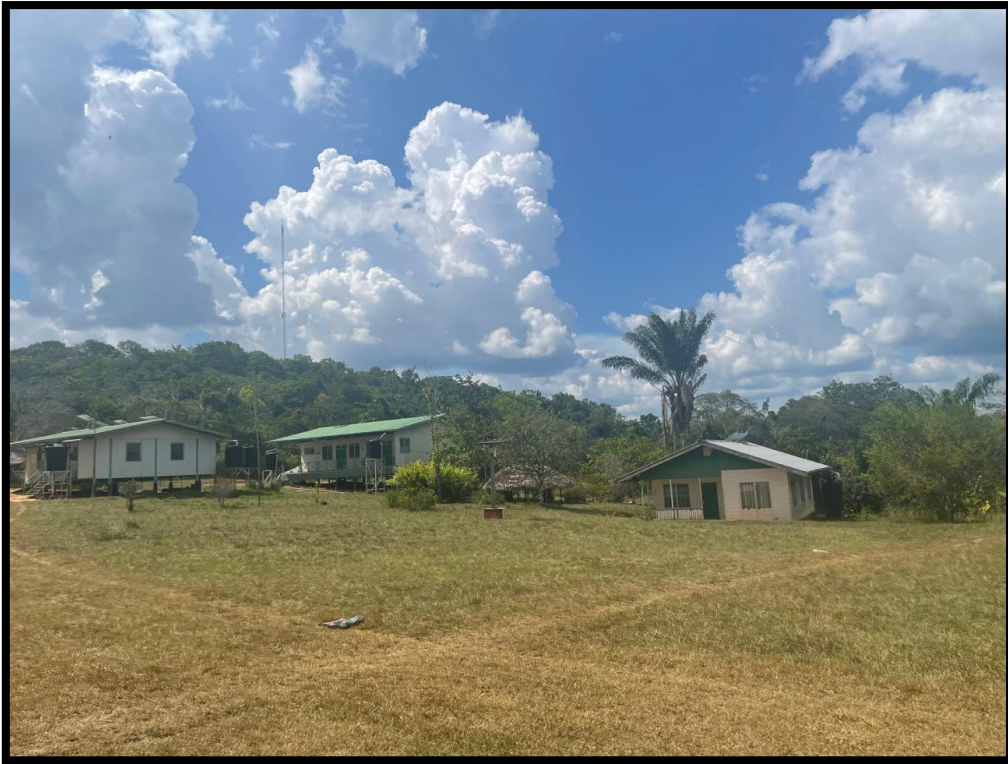
Figure 46. Traditional medicine health center located approx 50m from airstrip. Source: PlanEHS, 2024.
