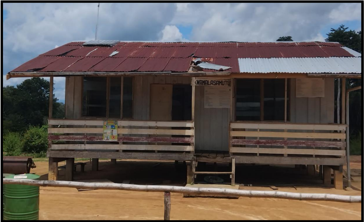
Figure 3. Current Station building from the outside. Source: Google, 2024.
