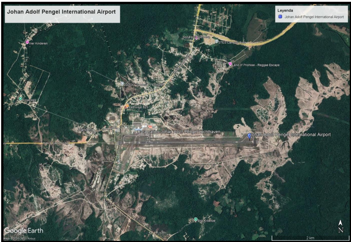
Figure 8. Johan Adolf Pengel International Airport. Source: Google Earth, 2024.
