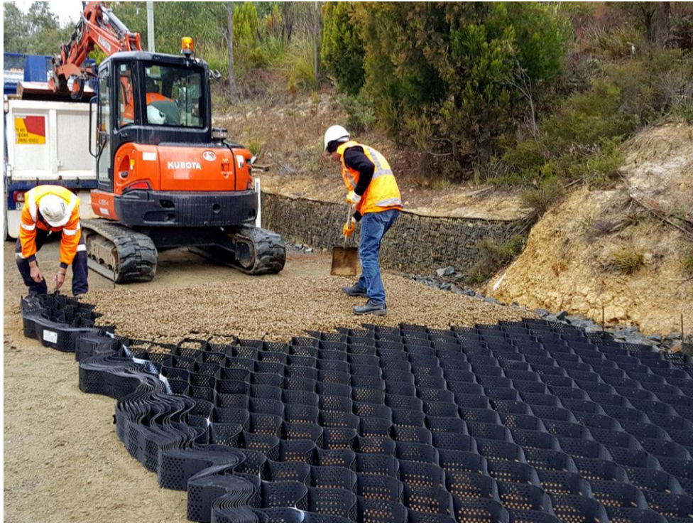
Figure 16: Impression of Geoweb installation.
