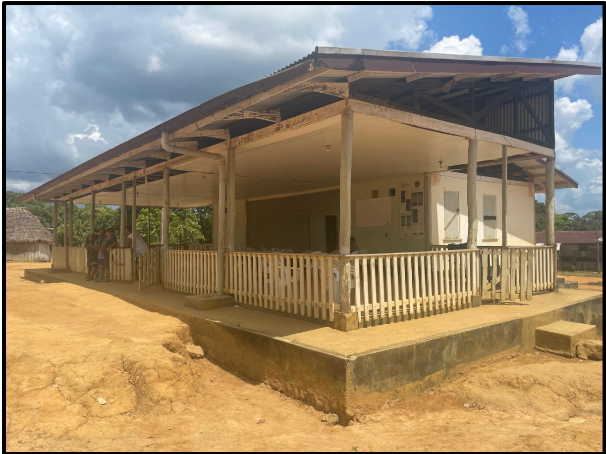
Figure 9 Building for institutional meetings
