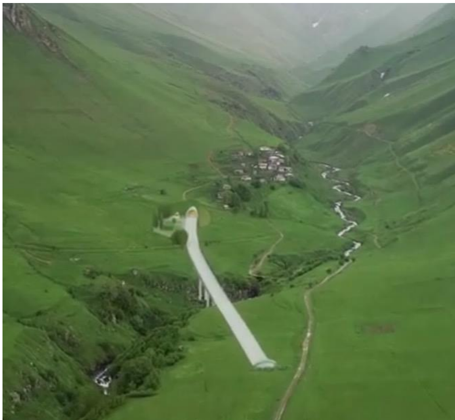
Figure 11: Tskere, Focus on cut and covers and portal of the long tunnel
