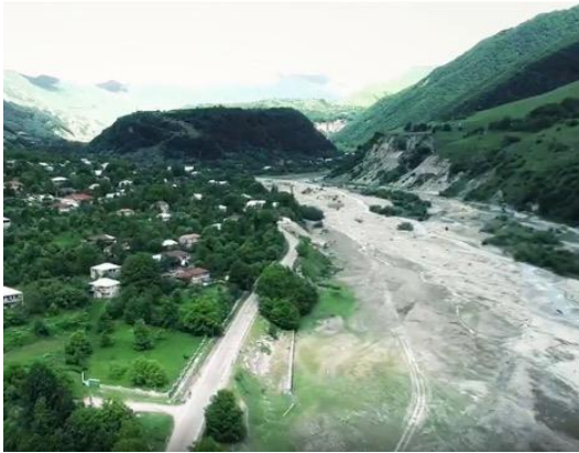
Figure 3: Kvesheti, Existing situation, East – West view
