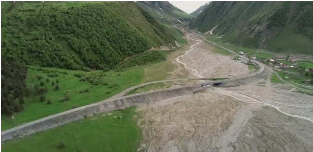
Figure 12: Kobi, Existing Situation
