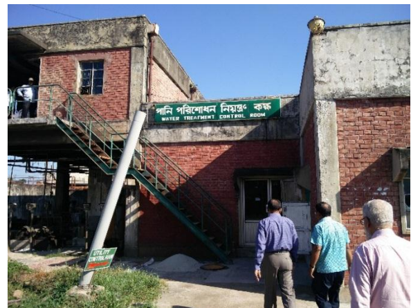
Water Treatment Plant Visit
