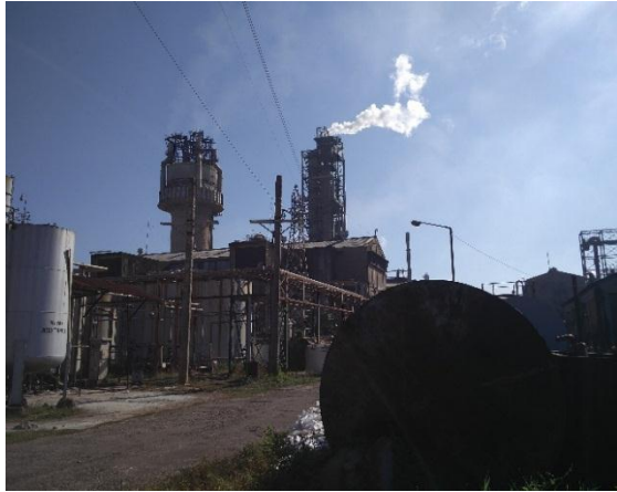
Chimney of Urea Fertilizer Factory
