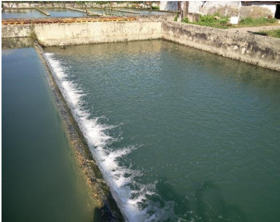
Clarified Water for Plant Use
