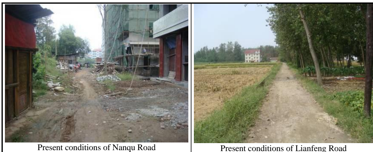
Fig. 5.7-1: Pictures of the Present Conditions of Some Roads for This Project
