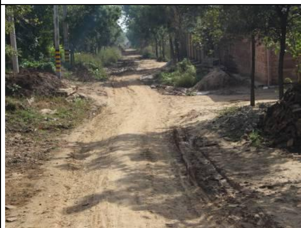
Present conditions of North Chuangye Road
