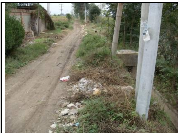
Present conditions of the east section of Hongyao Road
