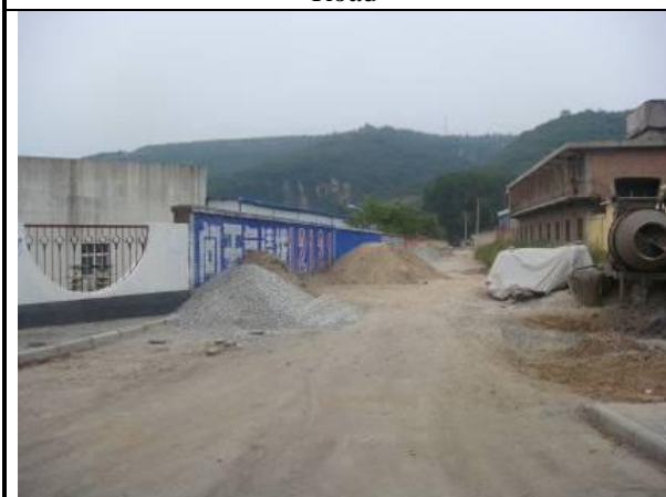
Present conditions of Wei'er Road
