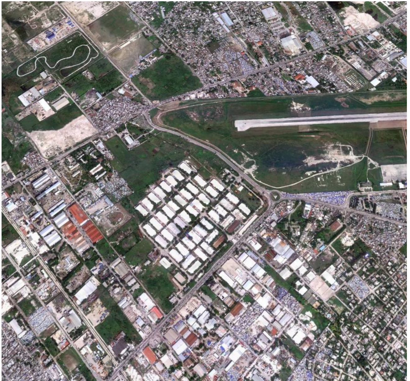
Figure 4 – SONAPI Industrial Park surrounding area
