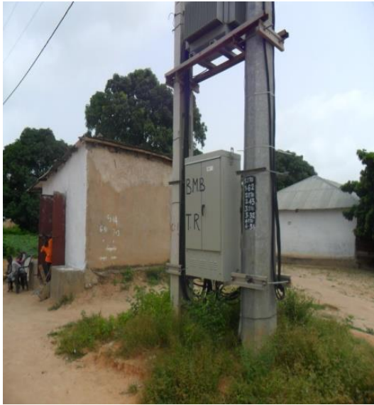
Figure 3: Electric poles with transformer near residential and commercial activities
