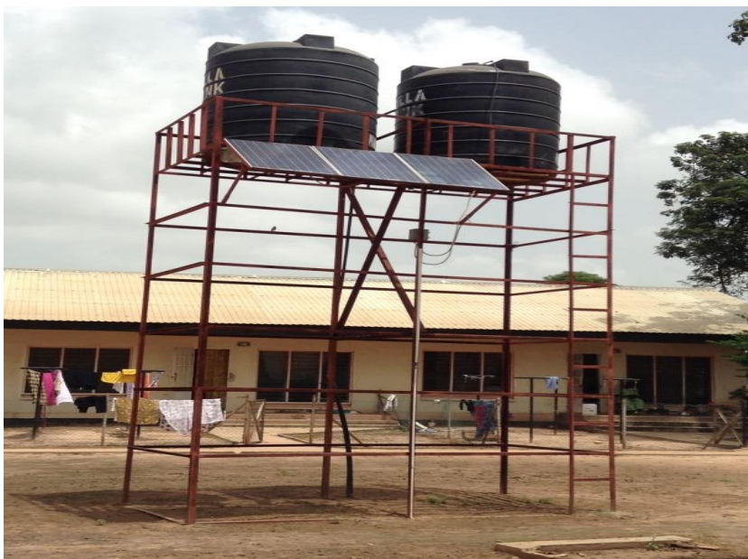
Non-operational solar panels for water pumping at Kuntair Health Centre
