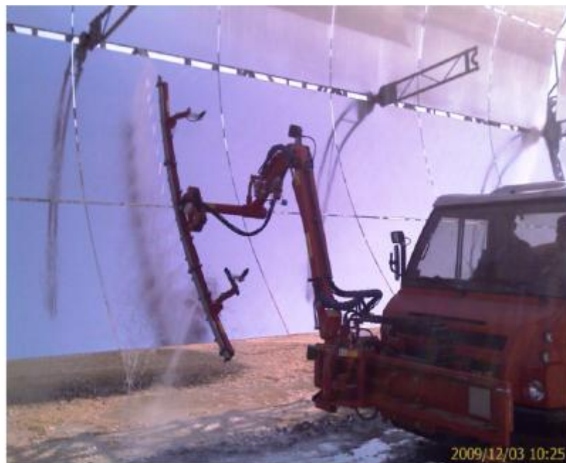
Figure12: The Washing Truck and Washing Operation
