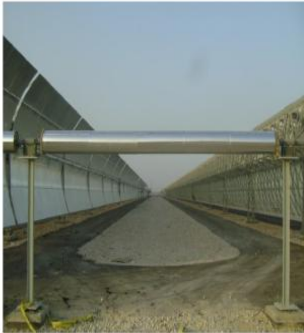
Figure 11: The Complete Loop with Insulation Works
