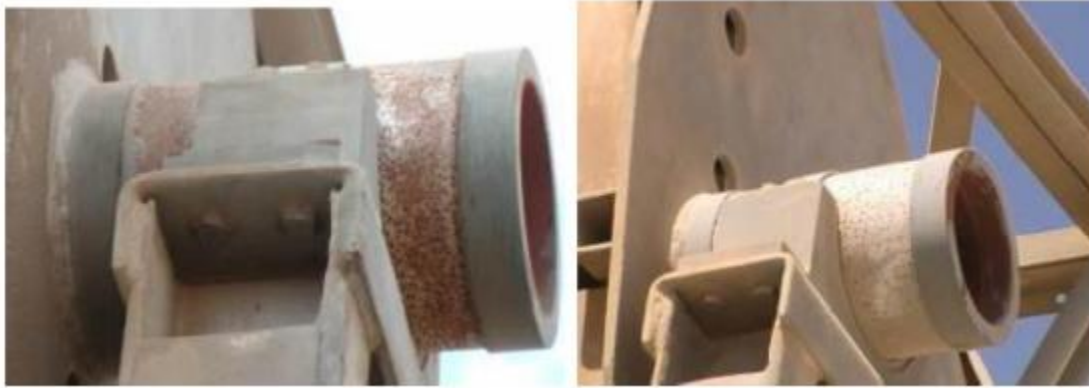
Figure 8: Pitting Occurred in Torque Tubes of the Collector
