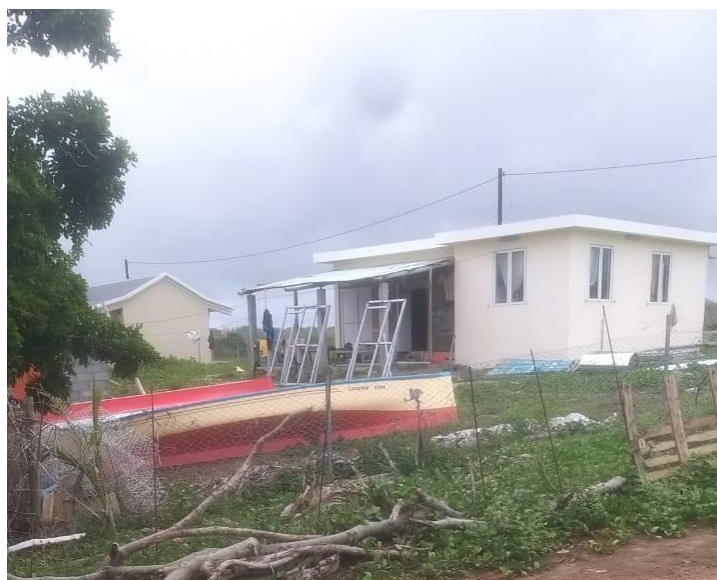
Figure 5: Relocated fishing warehouse in Les Salines
