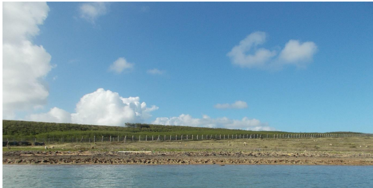
Figure 175: rocky coast in the west backfilled area
