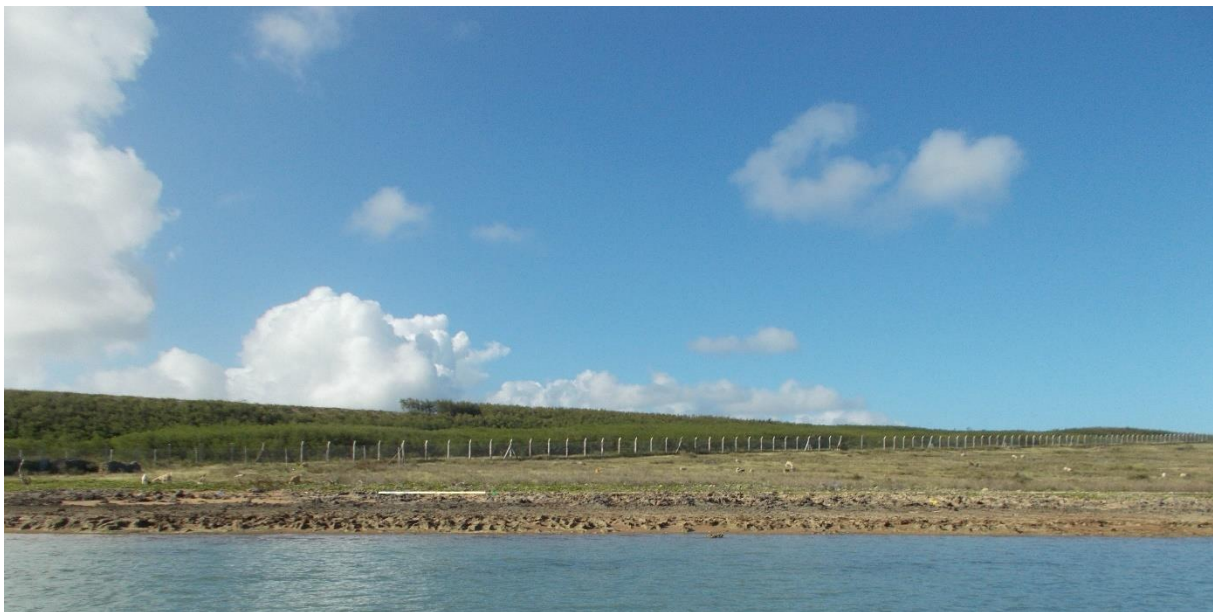
Figure 25: rocky coast in the west backfilled area
