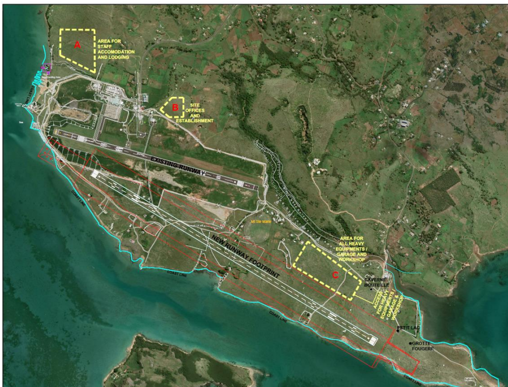
Figure 8: Temporary facilities associated with the construction phase
