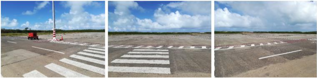
Figure 17: View of the existing drains observed around the apron in front of the passenger terminal building
