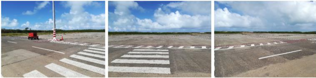
Figure 64: View of the existing drains observed around the apron in front of the passenger terminal building
