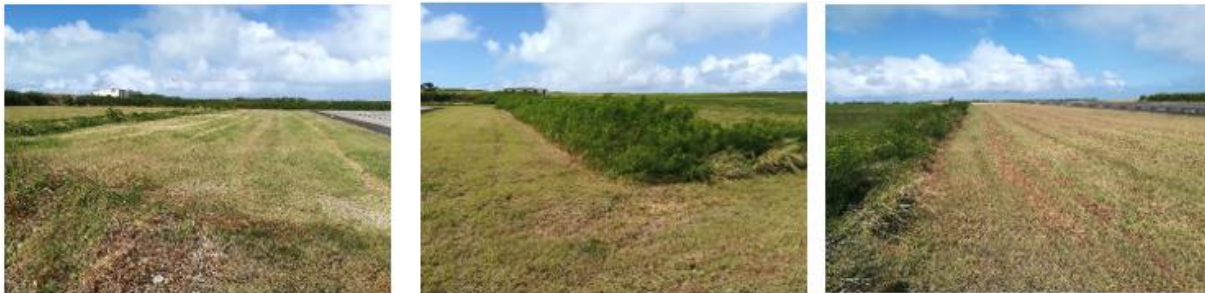
Figure 65: View of the existing drains observed around the apron in front of the passenger terminal building
