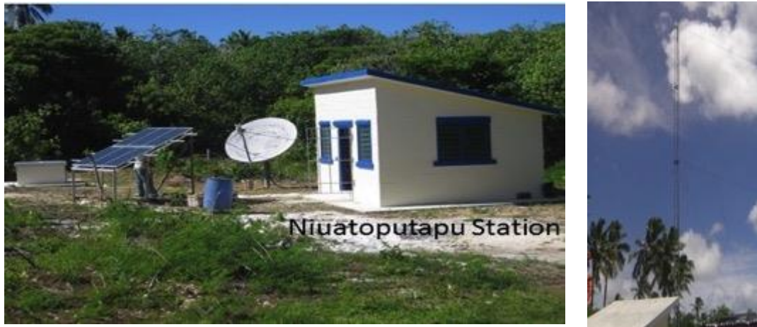
Figure 6 Existing Seismic Station infrastructure in Niuatoputapu and Tongatapu, Tonga
