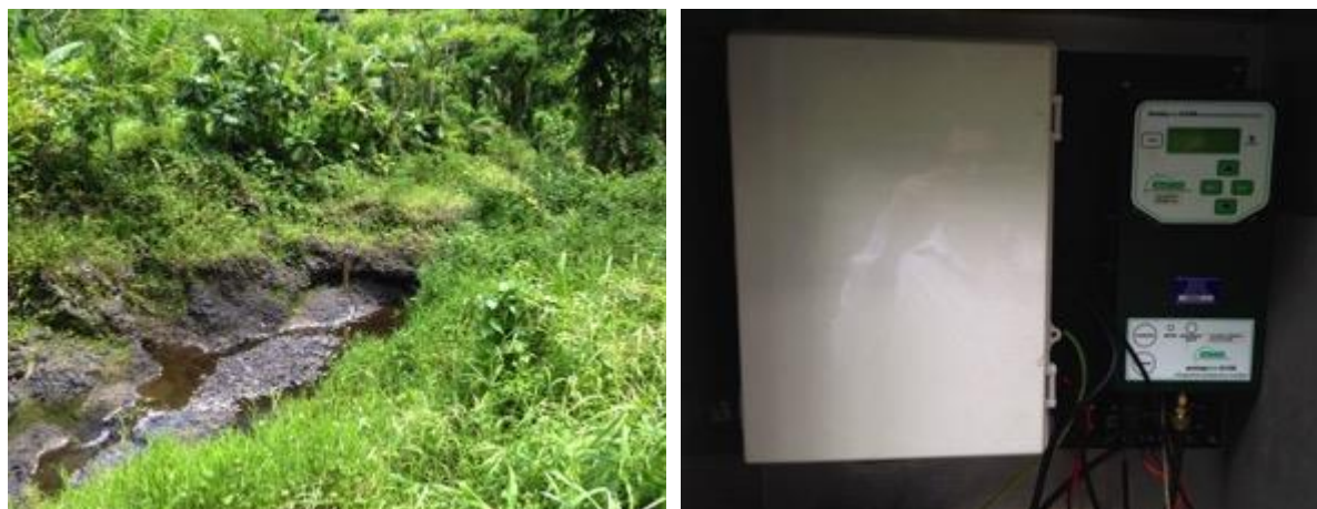
Figure 3 Hydrological monitoring station in Samoa
