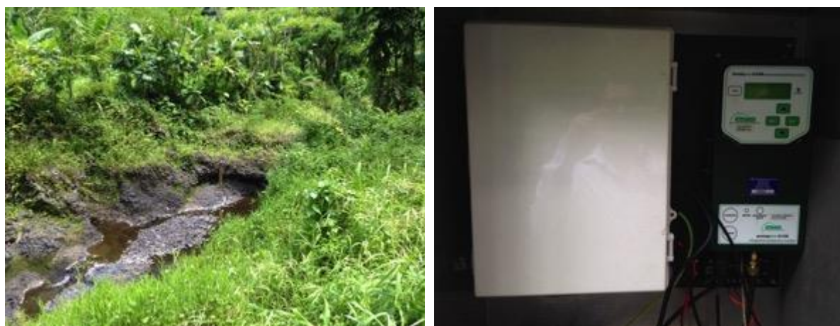
Figure 3 Hydrological monitoring station in Samoa
