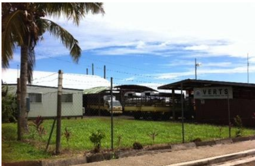
Figure 14 Existing block of land for NEOC office in Samoa
