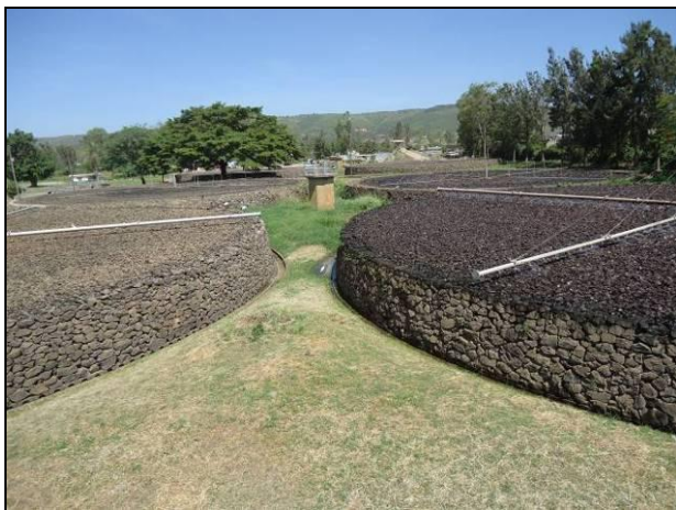
Trickling Filters
