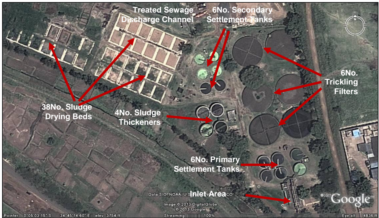
Kisat Conventional Treatment Plant
