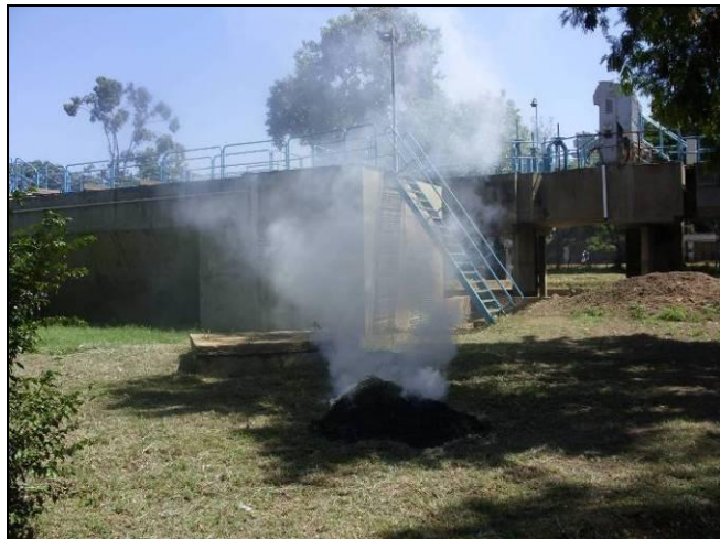
Open Air Burning of Wastes at Kisat Treatment Plant
