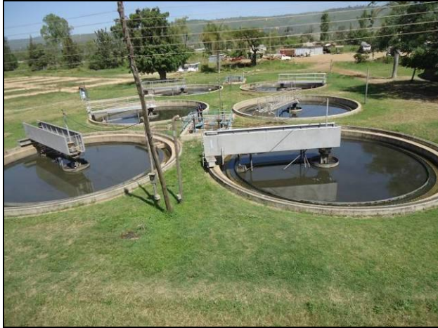
Secondary Settlement Tanks
