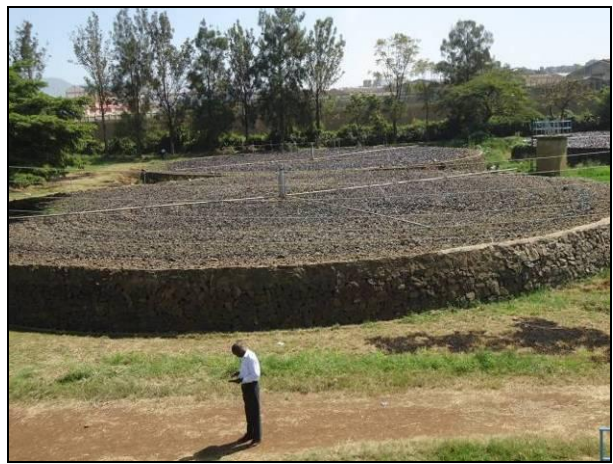
Trickling Filters
