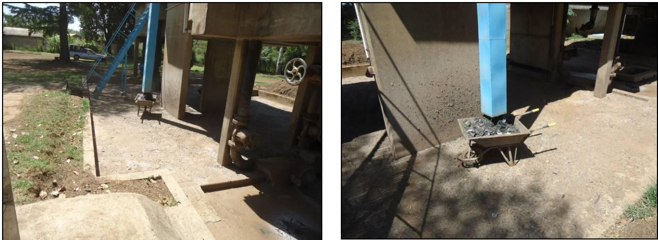
Grit Collection from Raw Sewage at the Reception Area
