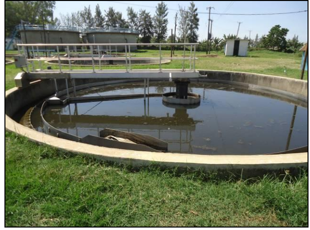
Secondary Settlement Tanks
