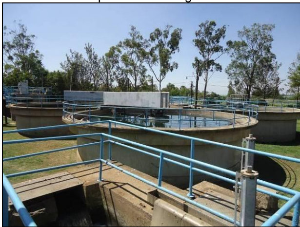
Primary Settlement Tanks
