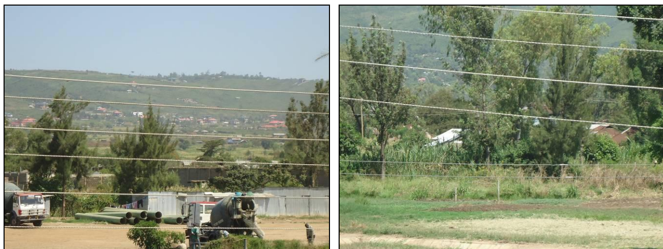
Figure 12: Settlements within Kisat Wastewater Treatment Plant
