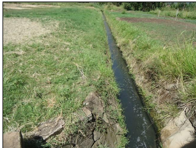
Treated Sewage Discharge Channle
