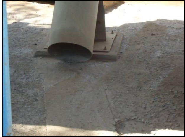
Overflow Raw Sewage Discharge at the Reception
