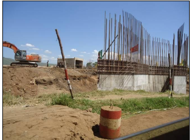
Ongoing Bypass Road Construction
