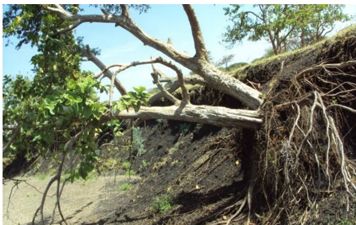
Figure 14: Eroded area along the Mongobakima river bank at the project area
