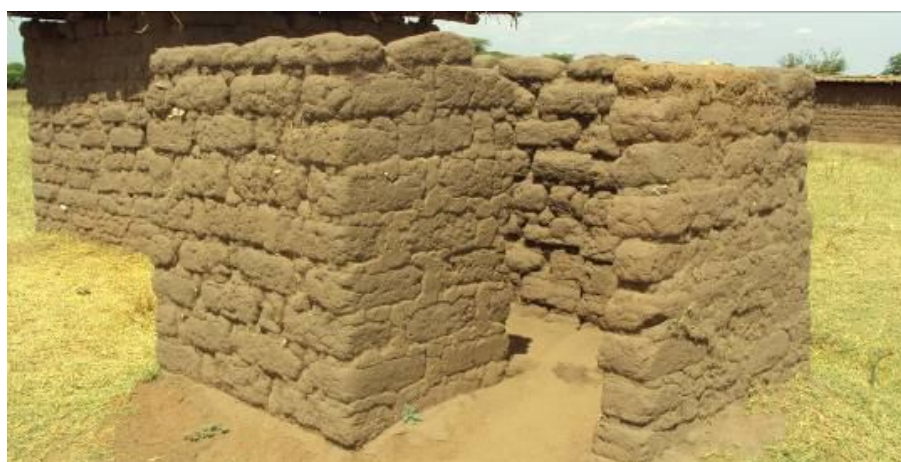
Figure 11: Type of common toilet at Mwabuma village
