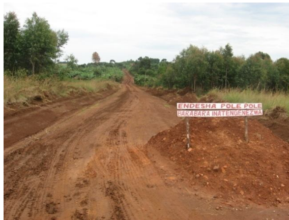
Figure 15: Road construction in progress near the project site warning drivers to reduce speed
