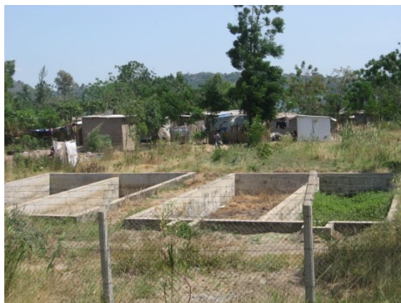
Figure 13: Properties located on the west side of the existing ponds to be affected by the project
