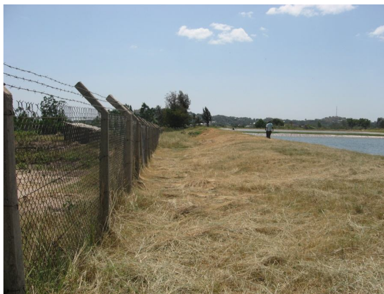
Figure 17: Fencing around the existing waste stabilization ponds
