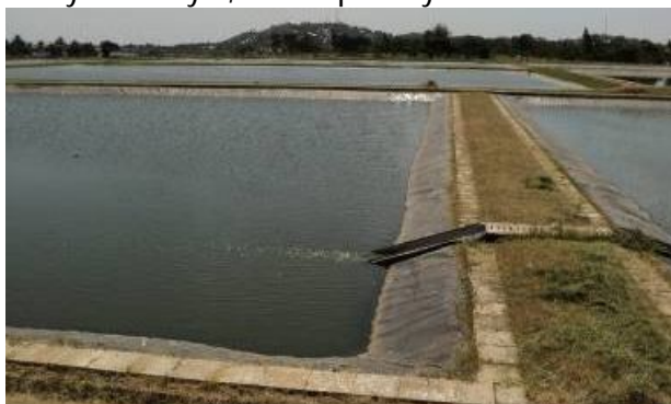
Figure 10: Waste Stabilization Ponds at Butuja- Ilemela
