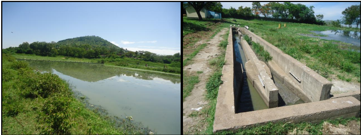
Figure 1 : Lagoon and water inlet at the sewage treatment, near the lake.
