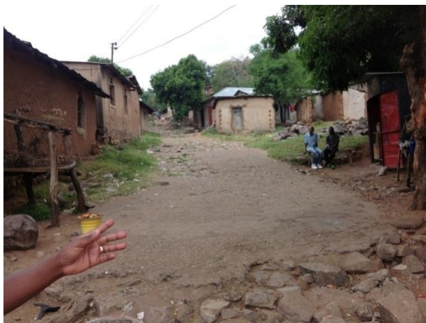
Figure 29: Disturbance to paved areas may leave this pavement demolished in Mabatini area
