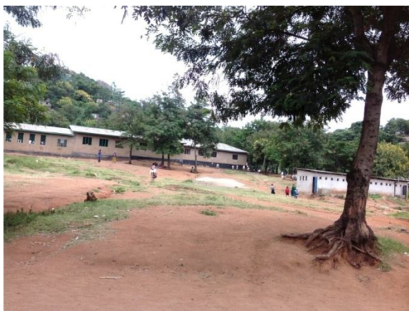
Figure 30: Pamba C Primary School which seem to have been let out of the sewerage system despite of being closer to the proposed sewerage system
