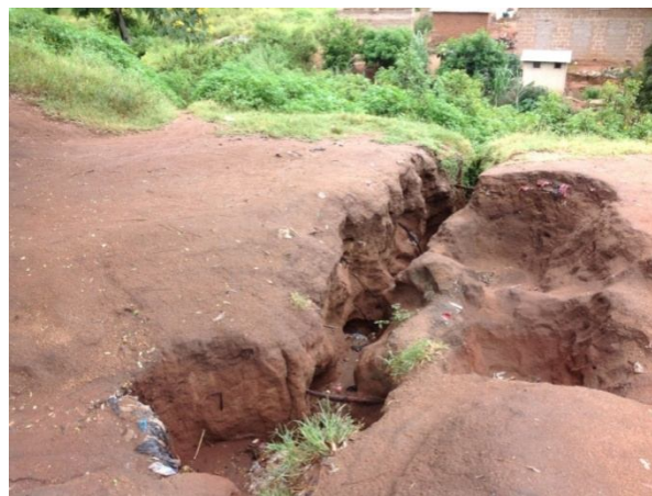
Figure 27: Soil erosion near Pamba C Primary School in Mabatini area
