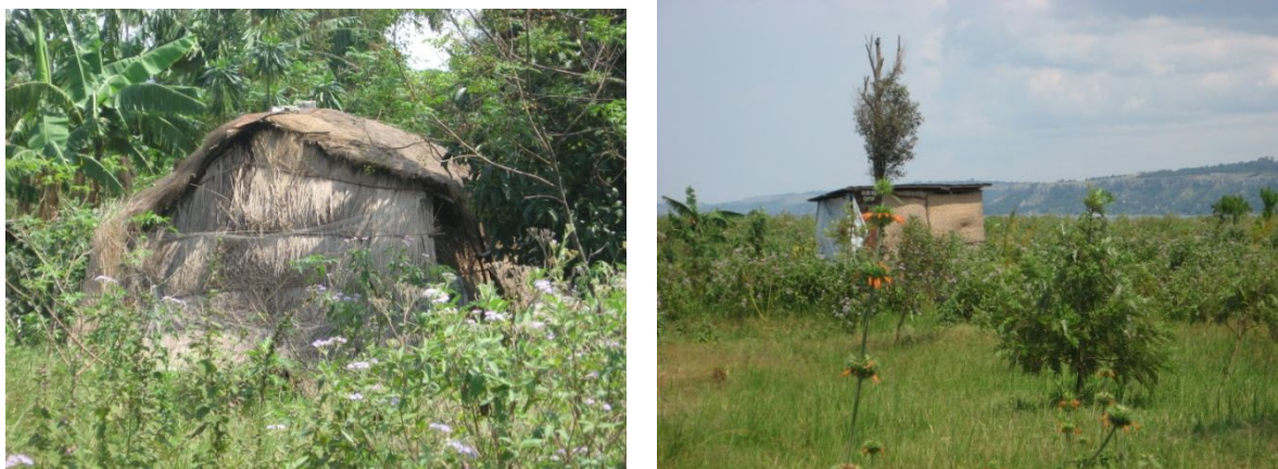
Figure 18: Some properties within the area earmarked for construction of waste stabilization ponds
