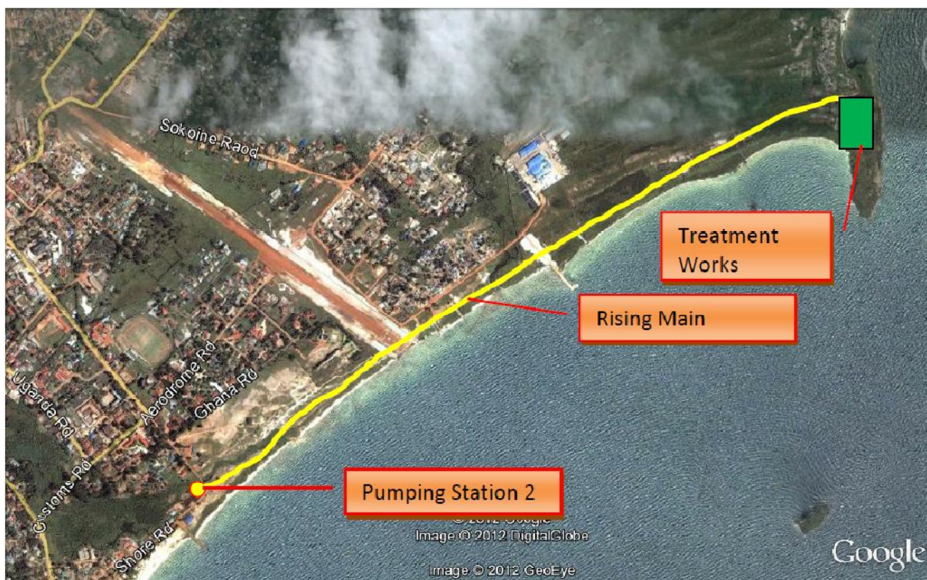
Figure 6: Satellite image showing the locations of the pump station, rising main and waste water treatment plant
