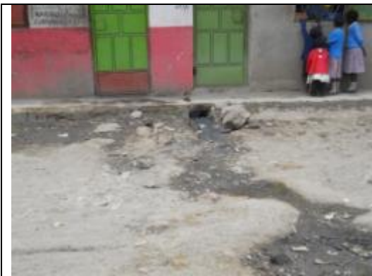
5. disposal of effluent into the road
