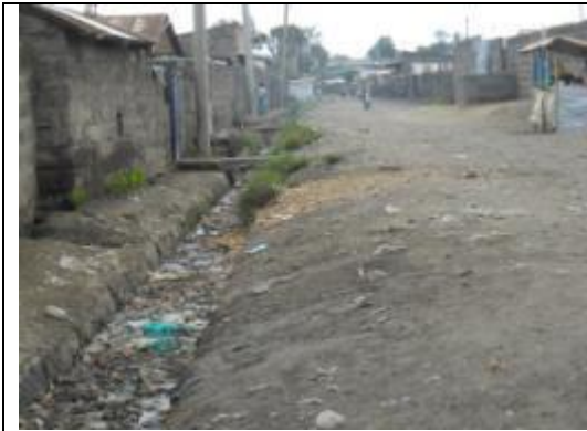
4 A blocked drainage
