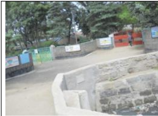
5. The drainage passing at the entrance of the two primary schools
