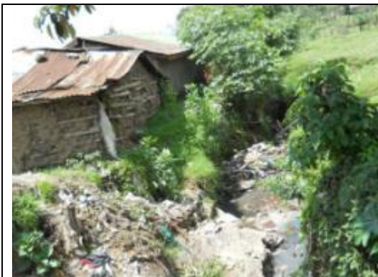
2. proposed drainage channel passes through a settlement in the lower end
