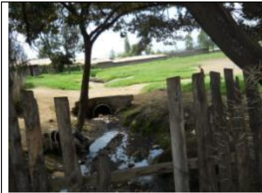
6..The drainage enters the school compound
