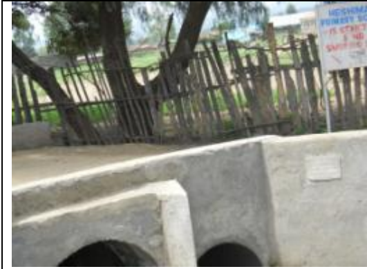
4. the drainage as it enters into the school compound
