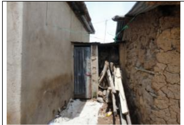
12..Toilets in makaburini slum
