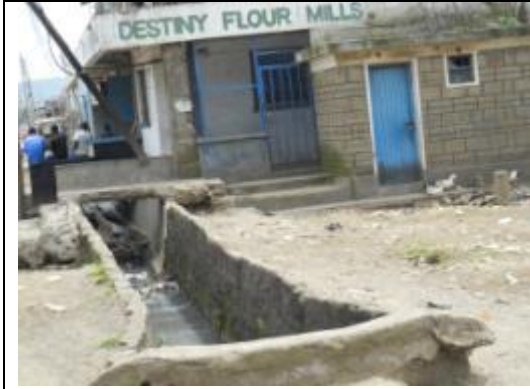
3. the drainage from the lower end
