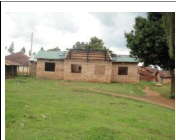
7This permanent house is being constructed right across a road reserve in Amalemba estate of Kakamega
