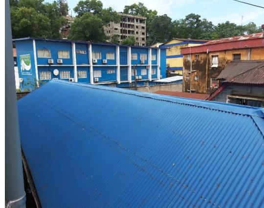
Plate 3: Stats SL Head Office Building-East Wing
