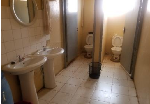
Plate 5: Male Wash Room (Ground Floor)
