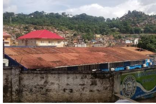
Plate 6: Asbestos Roof - To be Replaced and Disposed Off
