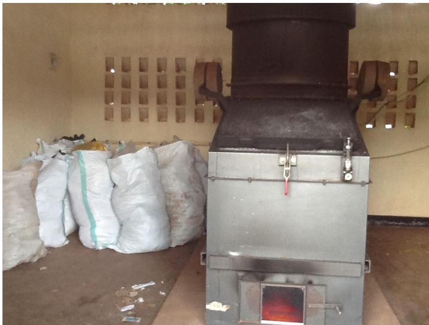
Waste storing and incinerator Kibungo District Hospital
