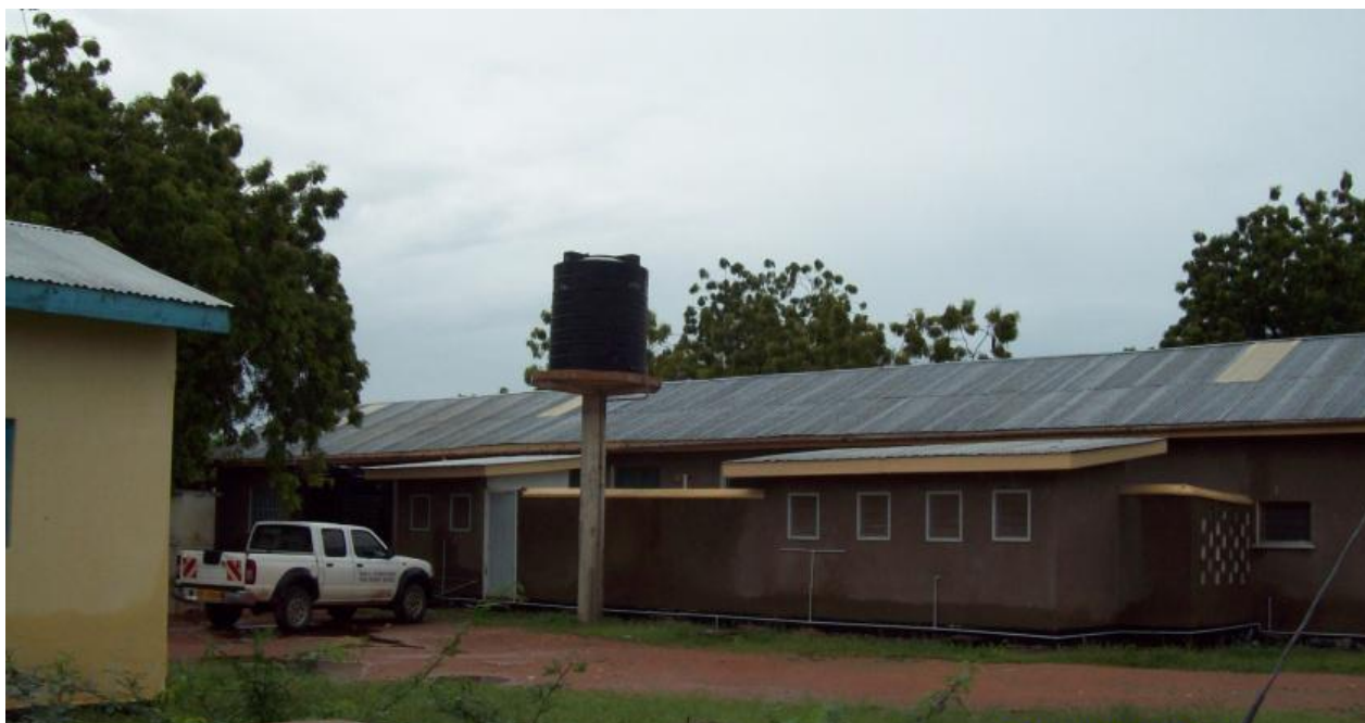
Figure 1: Part of Busia District Hospital
