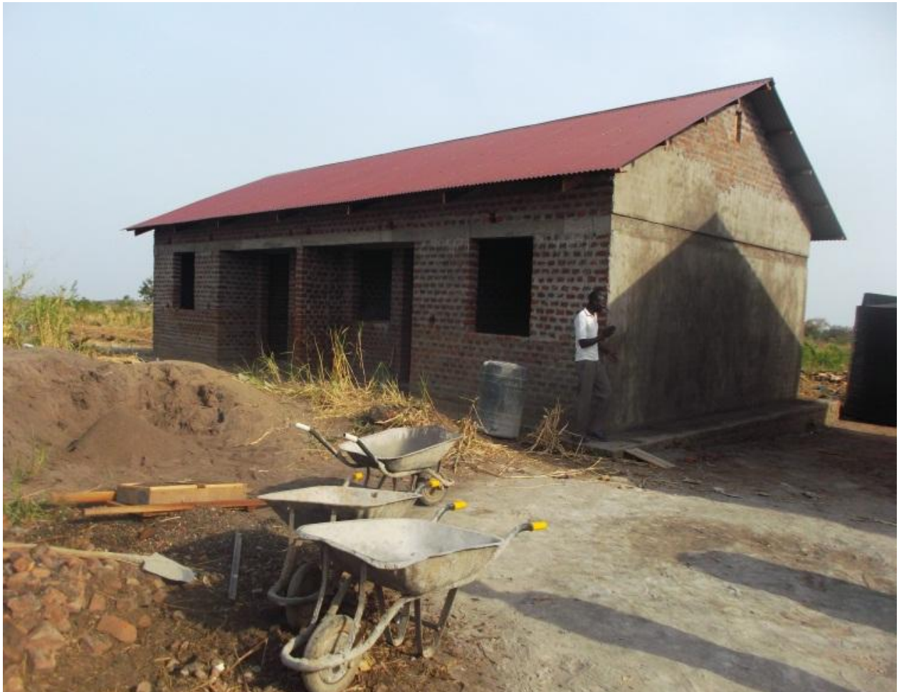
Figure 1: Staff quarters under constructed as part of NUSAF 2 at Nyamasoga P/S, Biiso S/C, Buliisa District
