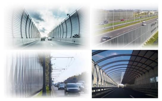
Figure 85. Examples of the shapes that noise barriers can take in attenuating noise from roads
