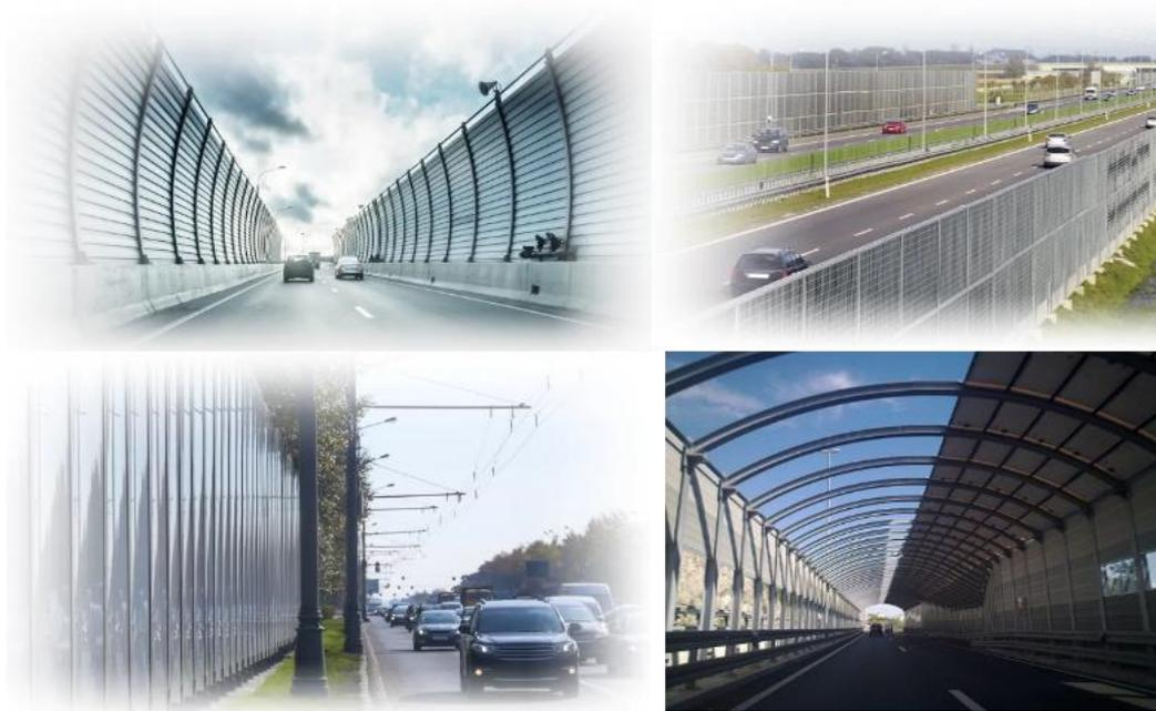
**Figure 85. Examples of the shapes that noise barriers can take in attenuating noise from roads**
