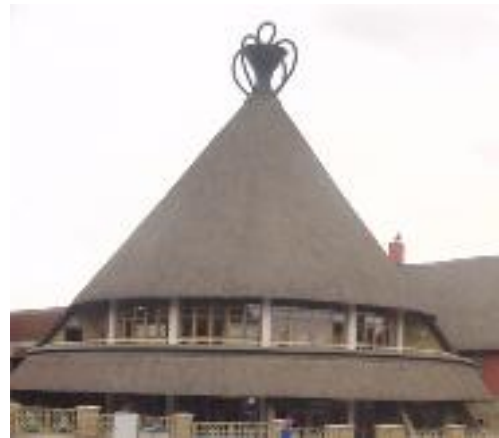
Image 2: The Basotho Hat (Mokorotlo) building
