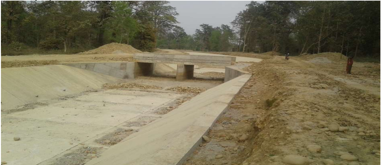
Figure 2-1: Canal crossing in the feeder canal constructed under MoRJKIS Phase I
