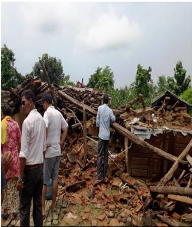
Damaged House by flood
