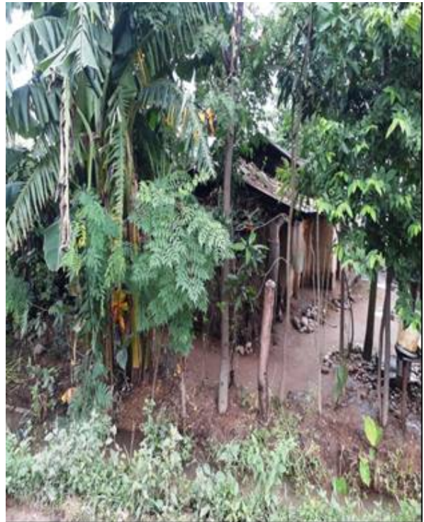
Flood Affected house at Bhagatpur, Jamara CA
