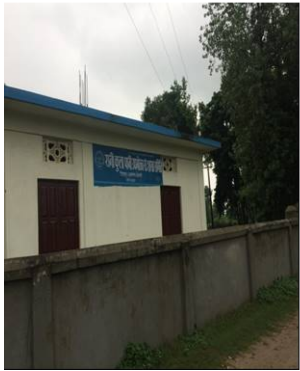
Office Building of Rani Kulo WUA
