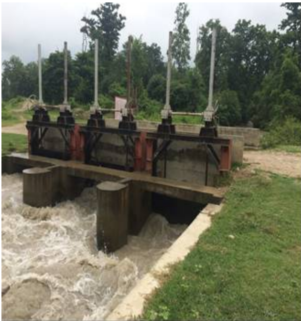
Water control system
