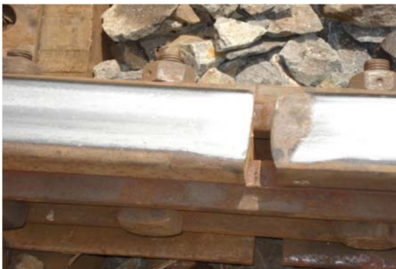
Several rails deformed at the joints or in poor condition, which can cause high dynamic forces when trains are passing
