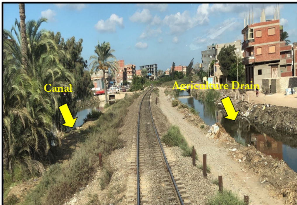
Figure 6-2: Construction of new railway track between two water bodies
