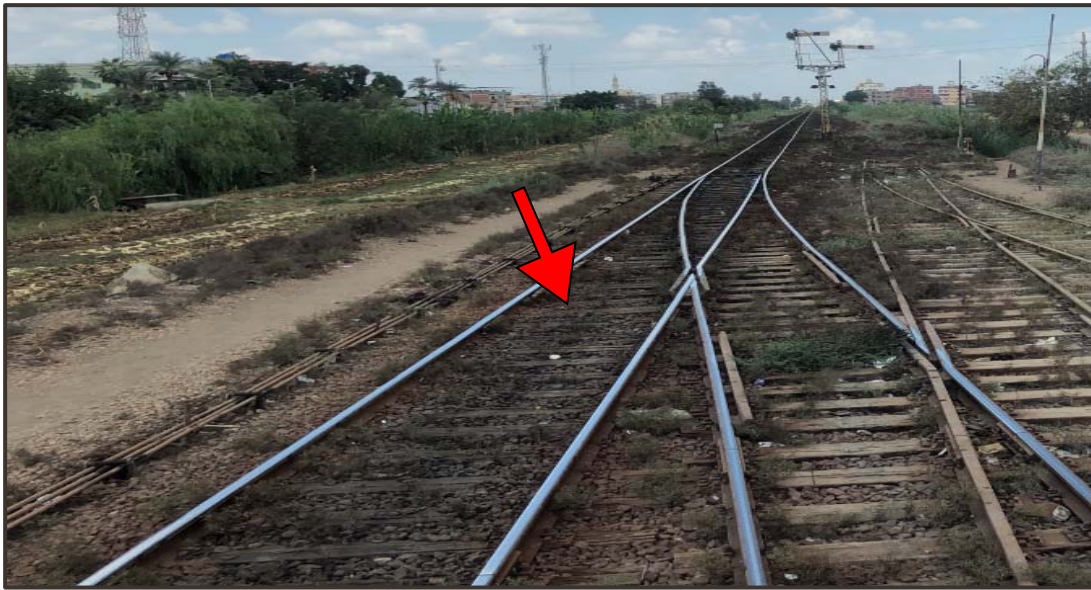
Figure 4-16: Contaminated wooden sleepers
