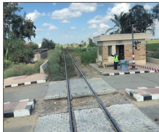
Developed Level Crossing
