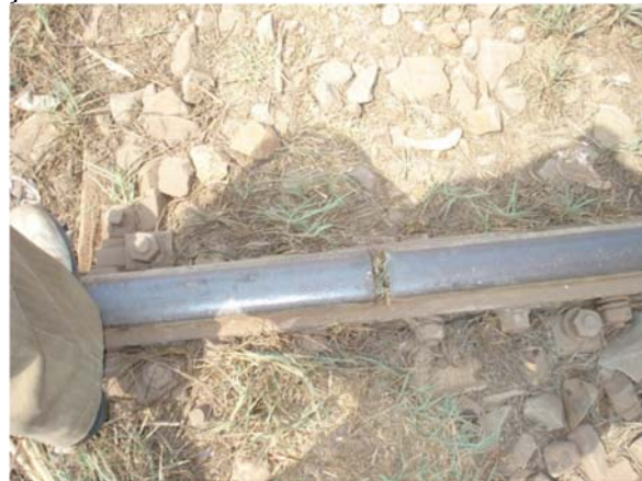
Several rail sections have not electrical continuity due to the gap at the joints, or the physical connection is in bad condition
