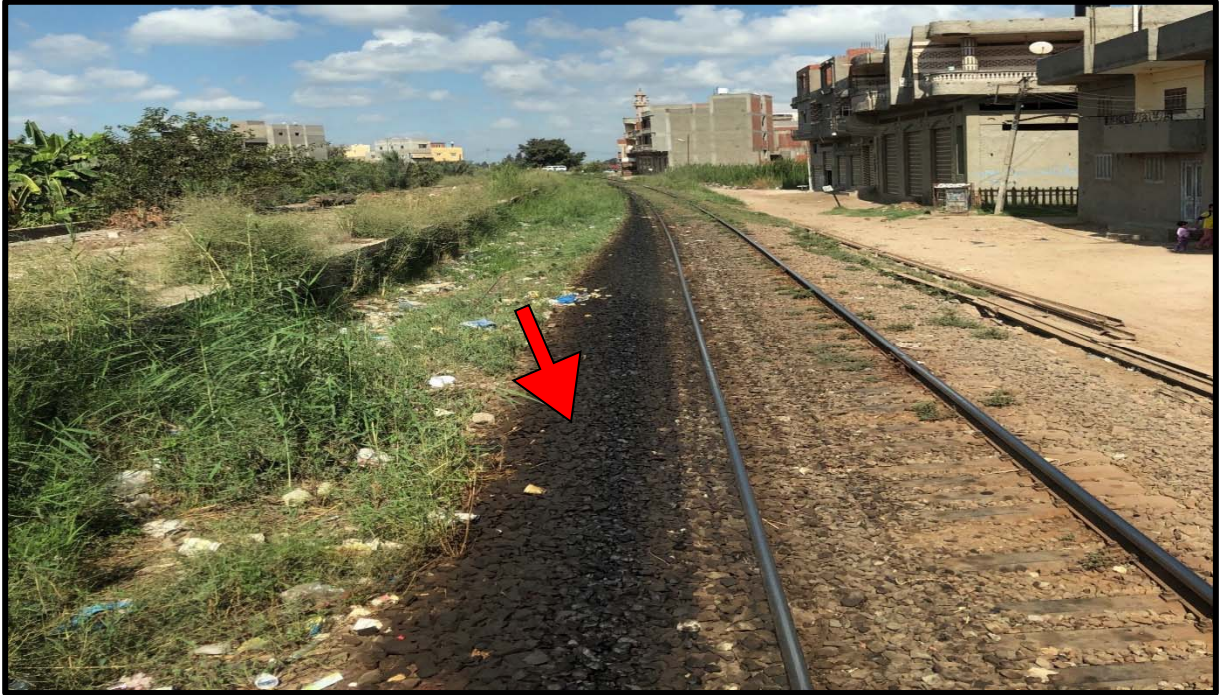
Figure 4-17: Oil spills observed near Ras El Khaleej station
