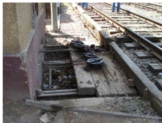
Signalling signals are controlled mechanically
