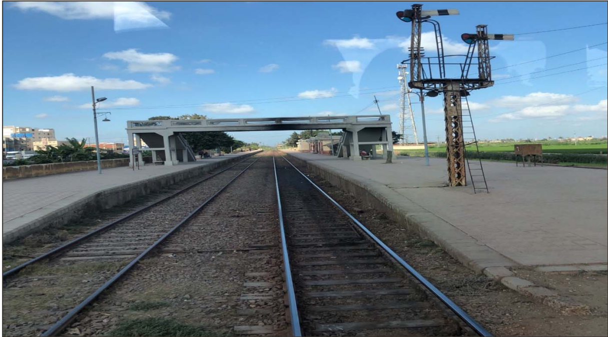
Figure 3-12: Kafr Saad station with double track
