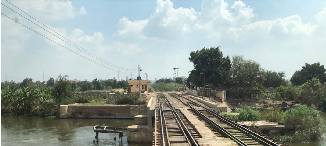
Figure 4-26: Trees and shrubs grows on canal banks
