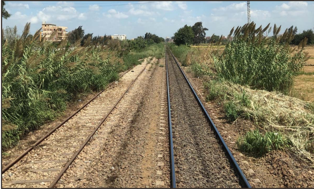
Figure 3-6: Railway Tracks ready for doubling
