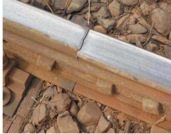
Bad condition of jointed track
