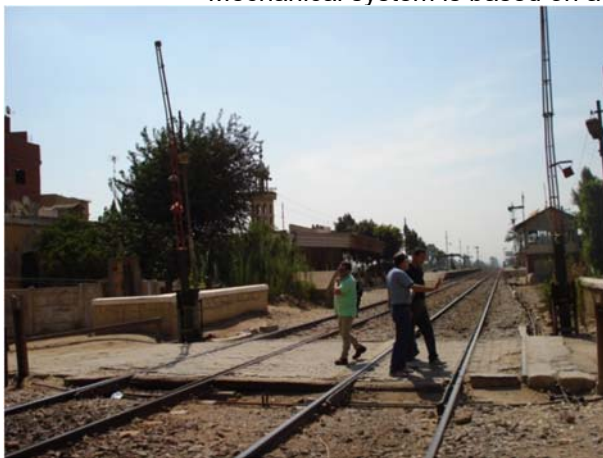
Local Control Panel (LCP) is controlled mechanically from BB and has a pavement where vehicles and people can use safely
