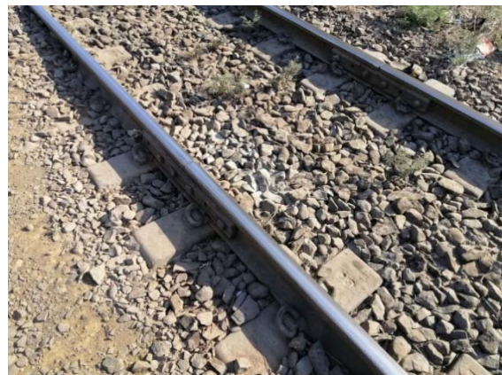
Twin block sleepers with Pandrol fasteners
