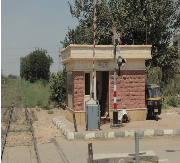
Upgraded Level crossing
