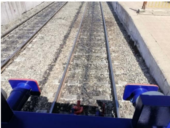
Mono block sleepers with Vossloh fasteners
