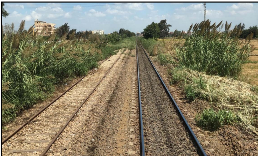
Figure 0-3: Railway Tracks ready for doubling
