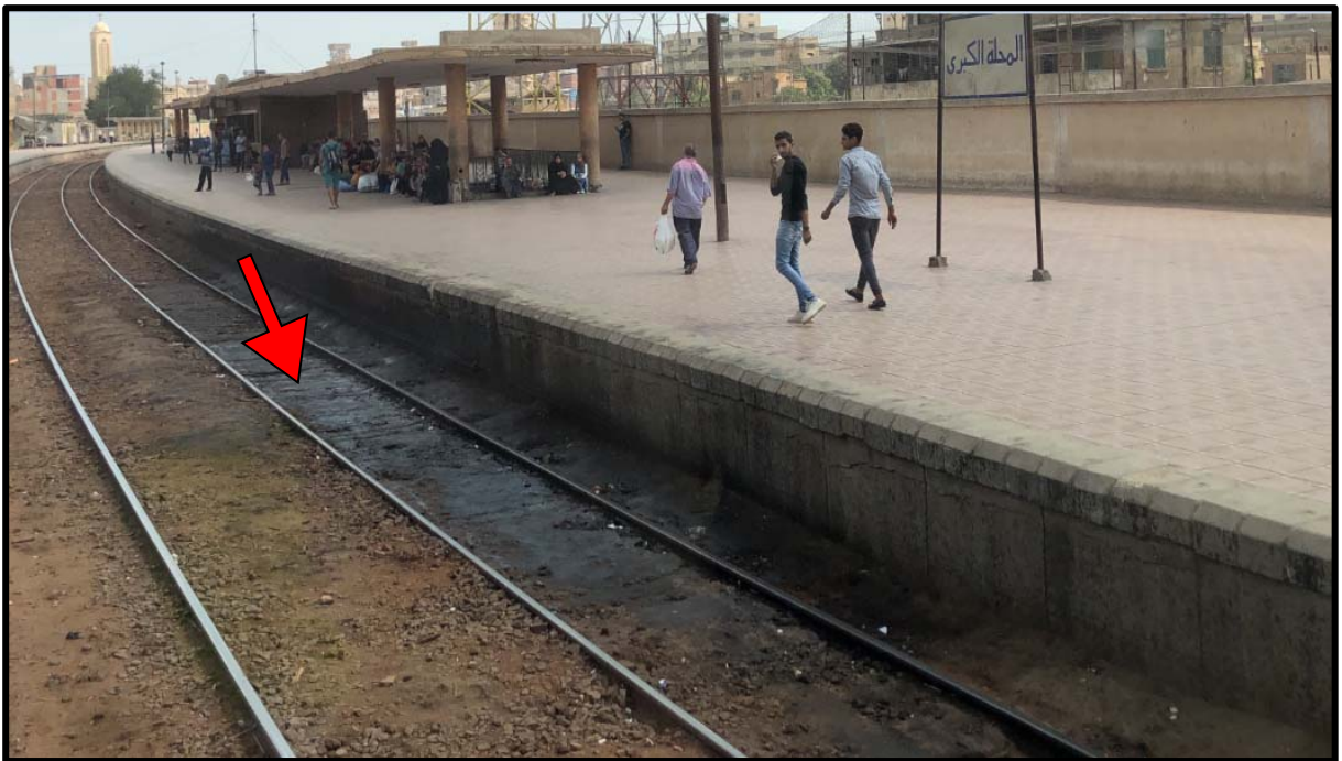
Figure 4-18: Spilled oil on the ground of the railway line (El Mahala El Kobra Station)
