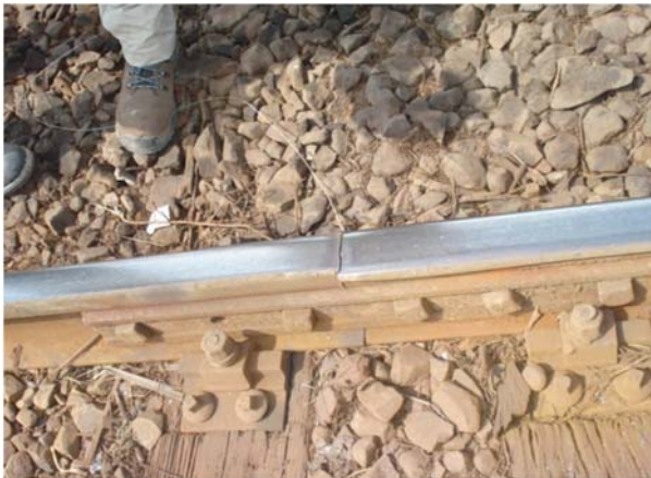
Several rail sections have not electrical continuity due to the gap at the joints, or the physical connection is in bad condition
