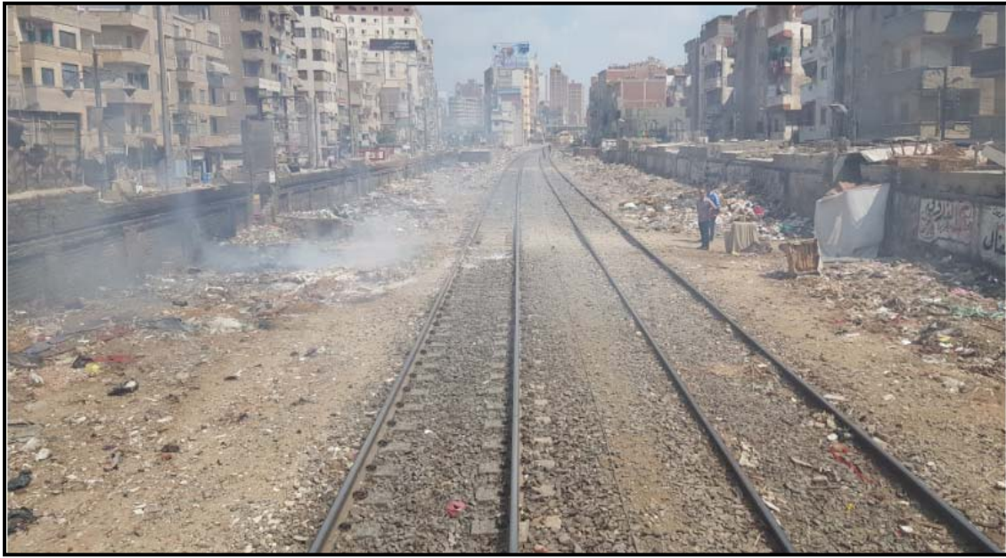
Figure 4-69 Open burnings of waste inside the railway corridor
