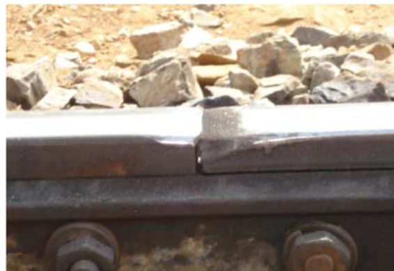
Several rails deformed at the joints or in poor condition, which can cause high dynamic forces when trains are passing
