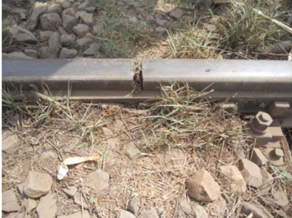
Bad condition of jointed track
