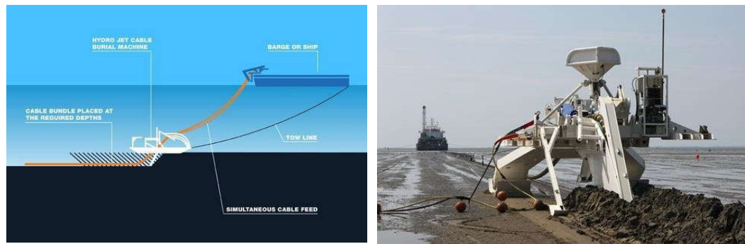
Figure 3.4. An example of submarine cable ploughs at sea and being towed from shore to deeper water by a cable laying ship
